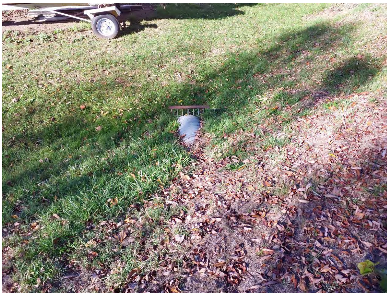
Figure 36: Entrance to culvert through berm on west side of Downstream Channel.
