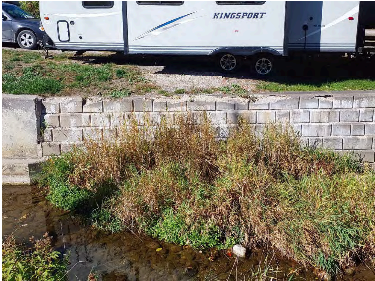
Figure 63: Excess sediment/ vegetation on the north side of the channel. Erosion of DuraHold blocks seen on top row.
