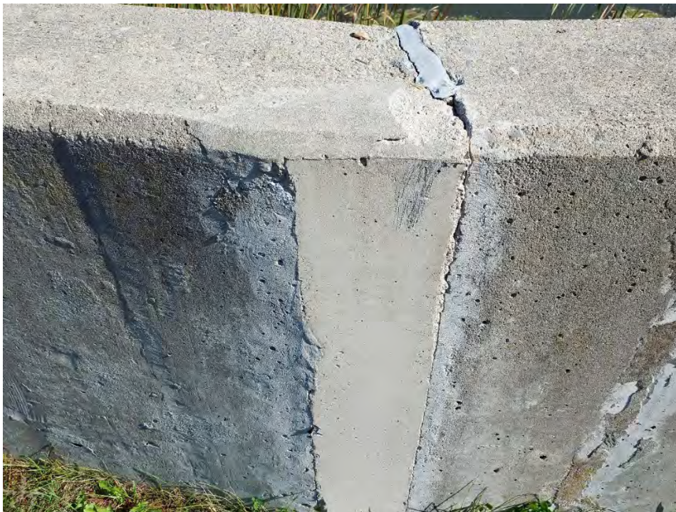
Figure 52: Roadside of concrete repair along Mill Street.
