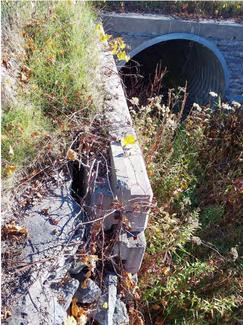
Figure 31:Wing wall (north side) downstream of the Double Arch culvert showing signs of separation.
