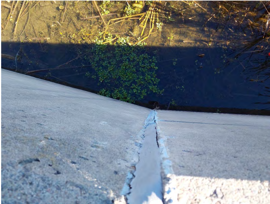
Figure 51: Repaired shifted concrete on west side of channel upstream of weir.
