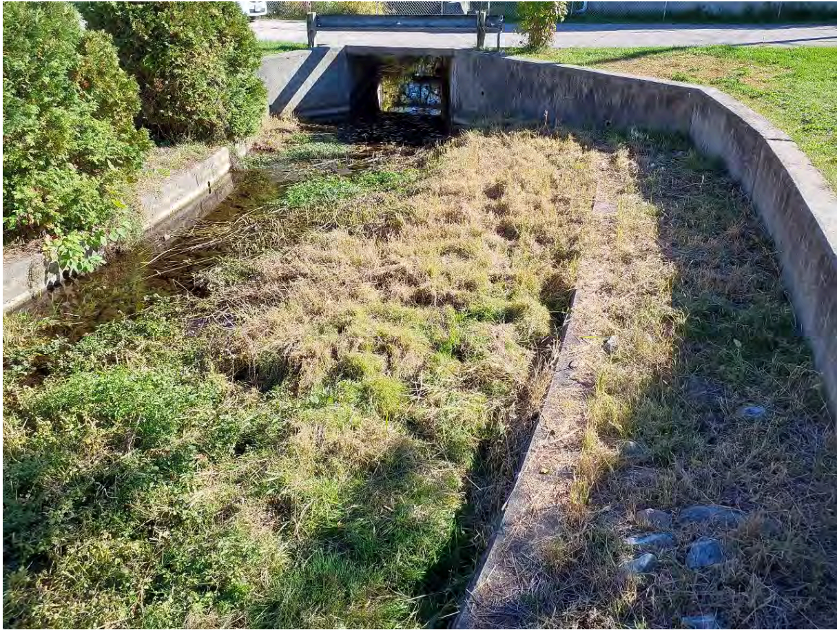
Figure 56: Channel crossing and vegetation within the flood channel adjacent to Park Street.
