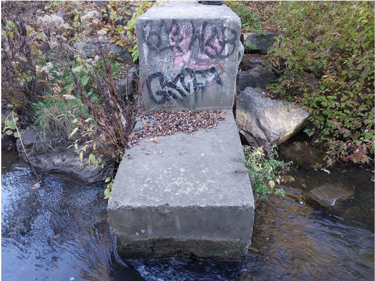
Figure 34: 2-Stage weir on north side of watercourse spalling along waterline.
