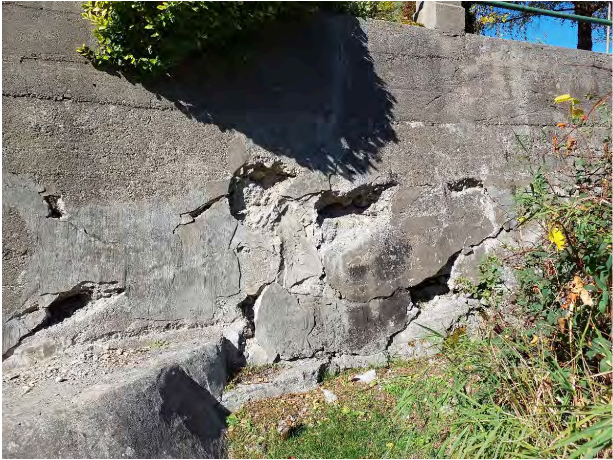
Figure 44: Large cracks and missing concrete along north side of Flood Channel, downstream of covered bridge.
