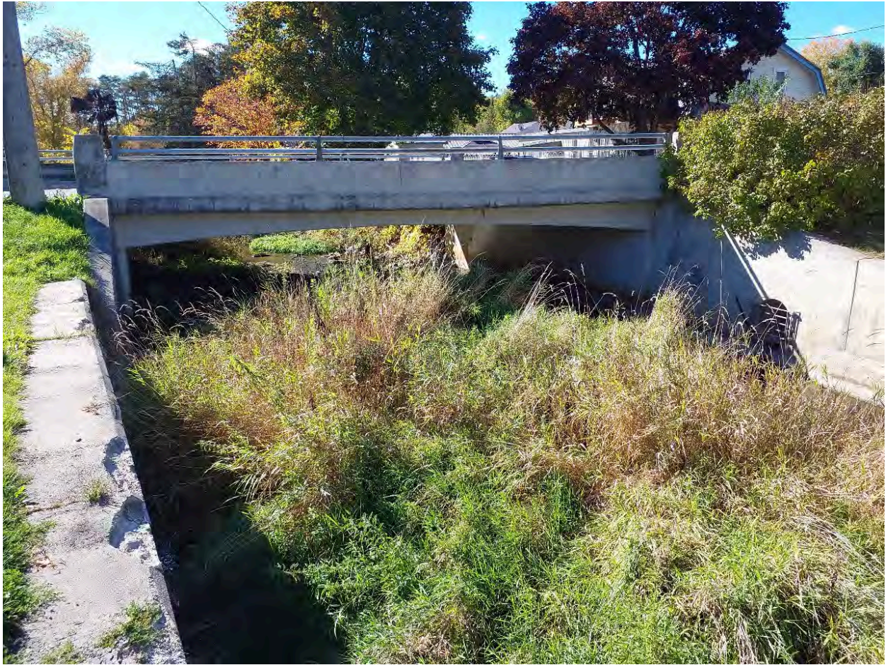
Figure 62: Excess sediment and vegetation downstream of the Simpson Street bridge within the channel. Photo taken facing upstream towards bridge.
