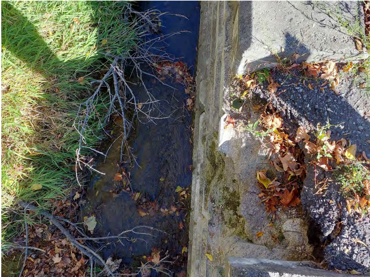
Figure 64:Erosion of DuraHold blocks downstream of Pellissier Street Bridge on south side where road drainage is located.
