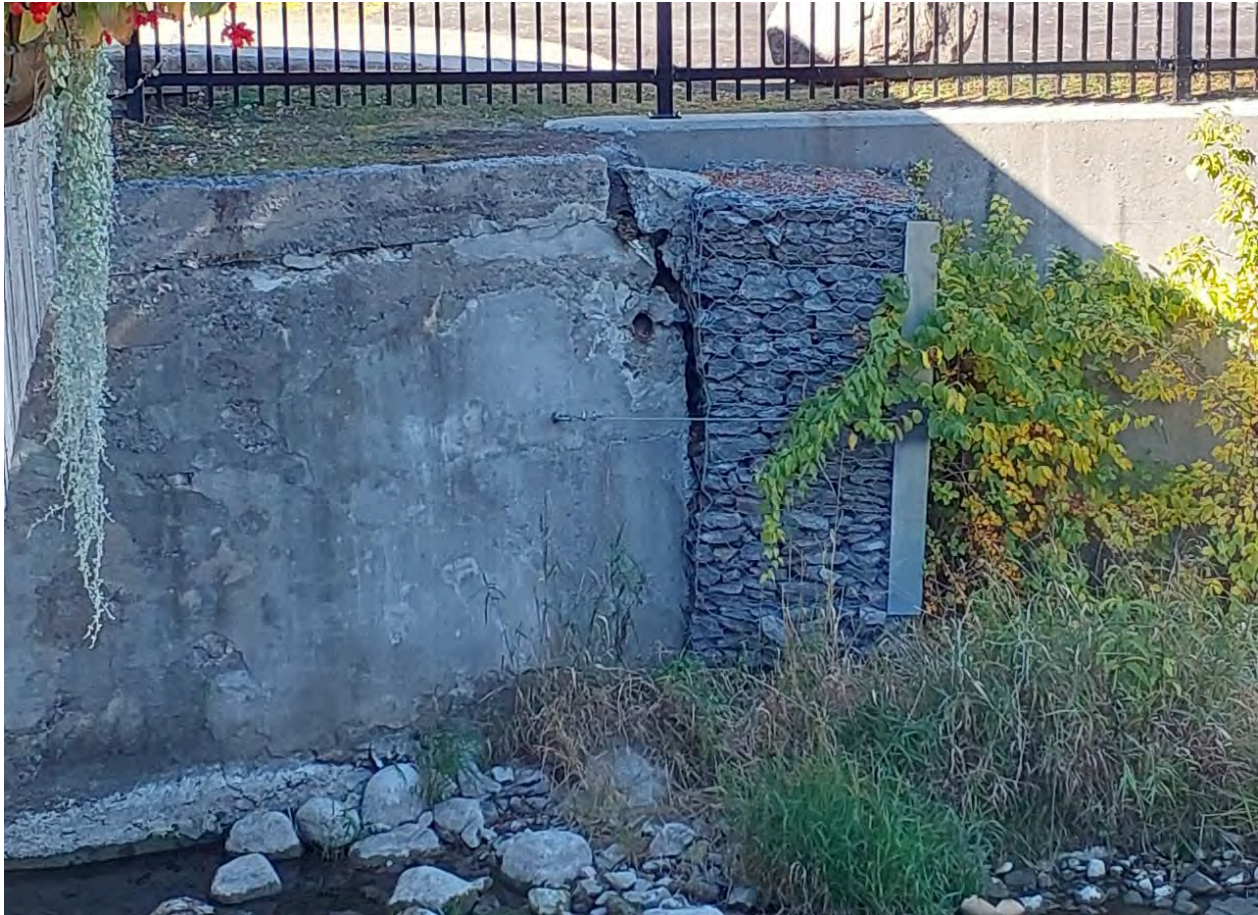
Figure 46: Repair work related to the gabion baskets pulling away from the concrete on the north side of the covered bridge.
