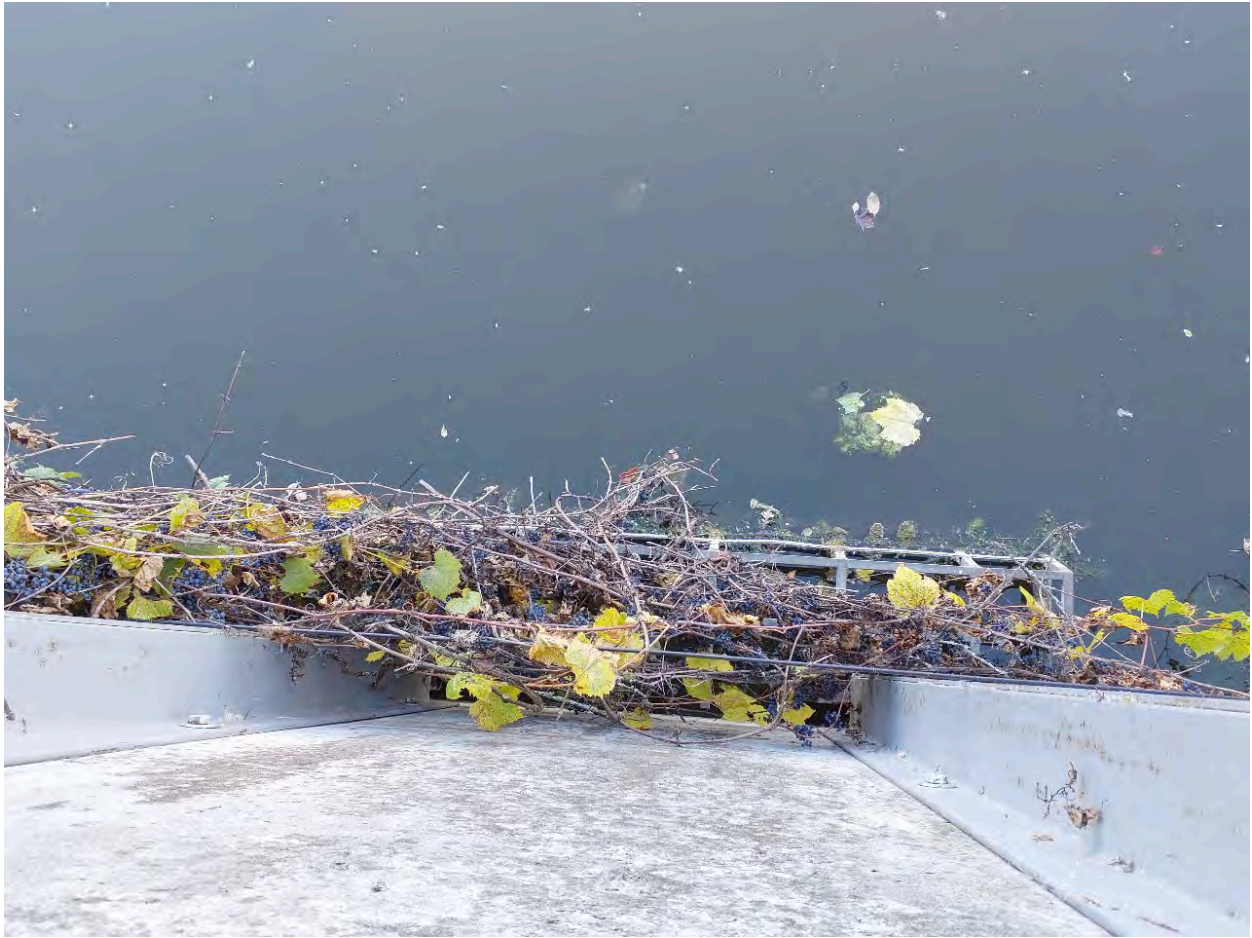
Figure 54: Top down view of vegetation impeding gate operation.
