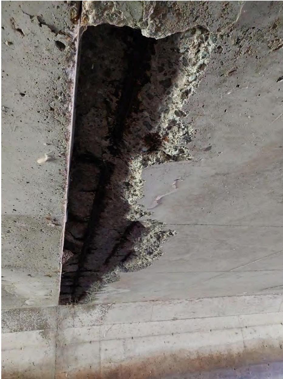
Figure 26: Roof of box culvert with exposed rebar under Foster Stearns Road box culvert.
