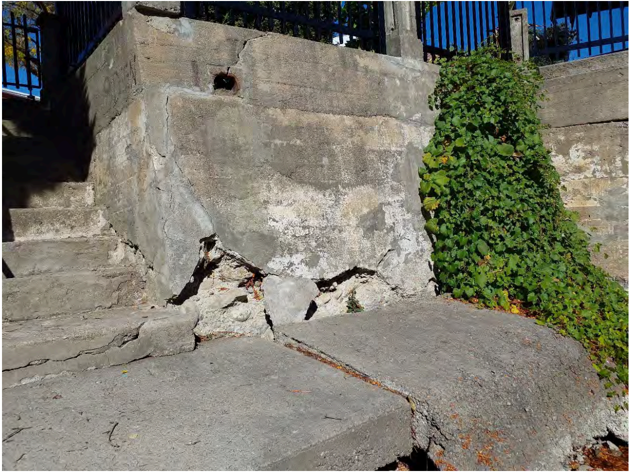
Figure 45: Large pieces of missing concrete along north side of Flood Channel, downstream of covered bridge.
