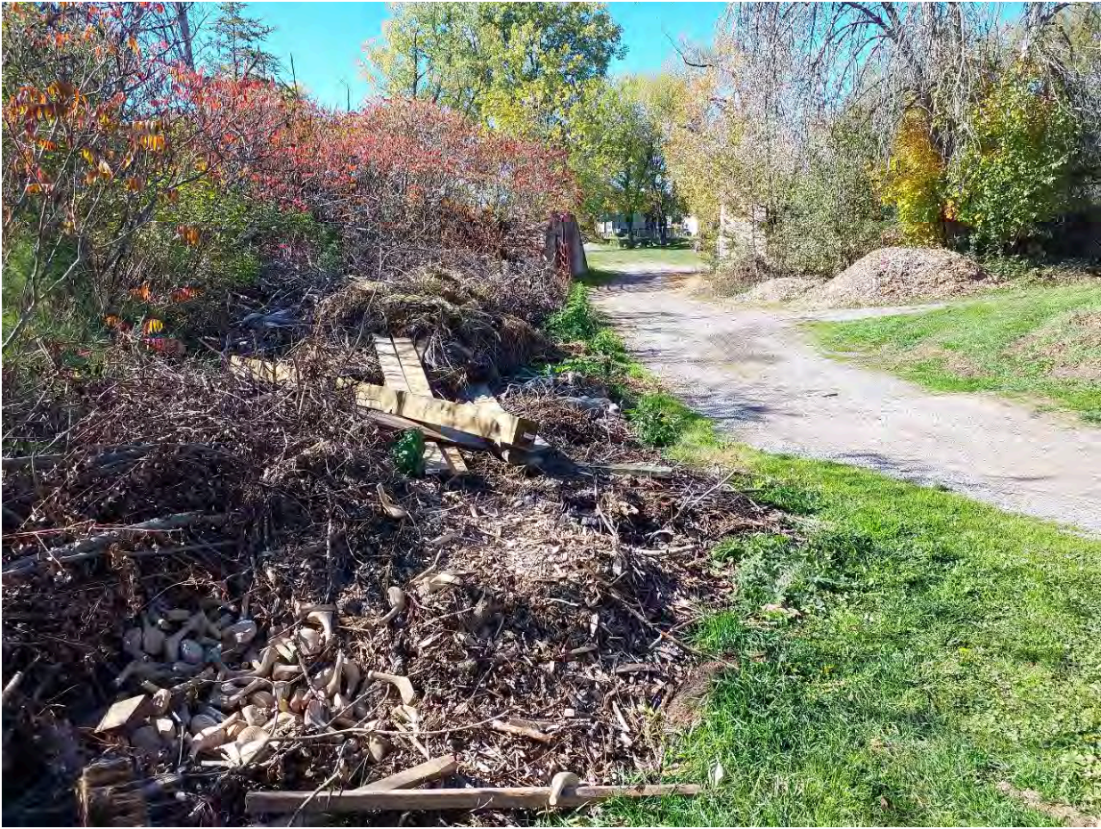
Figure 14: Debris within flood spillway east of golf course and berm
