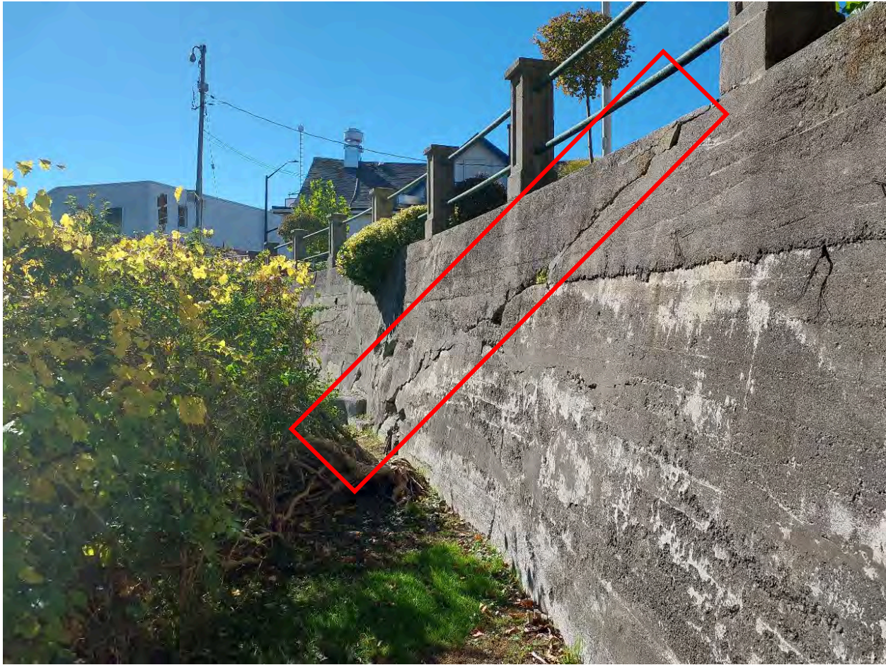
Figure 42: Cracks identified on north side of channel downstream of covered bridge
