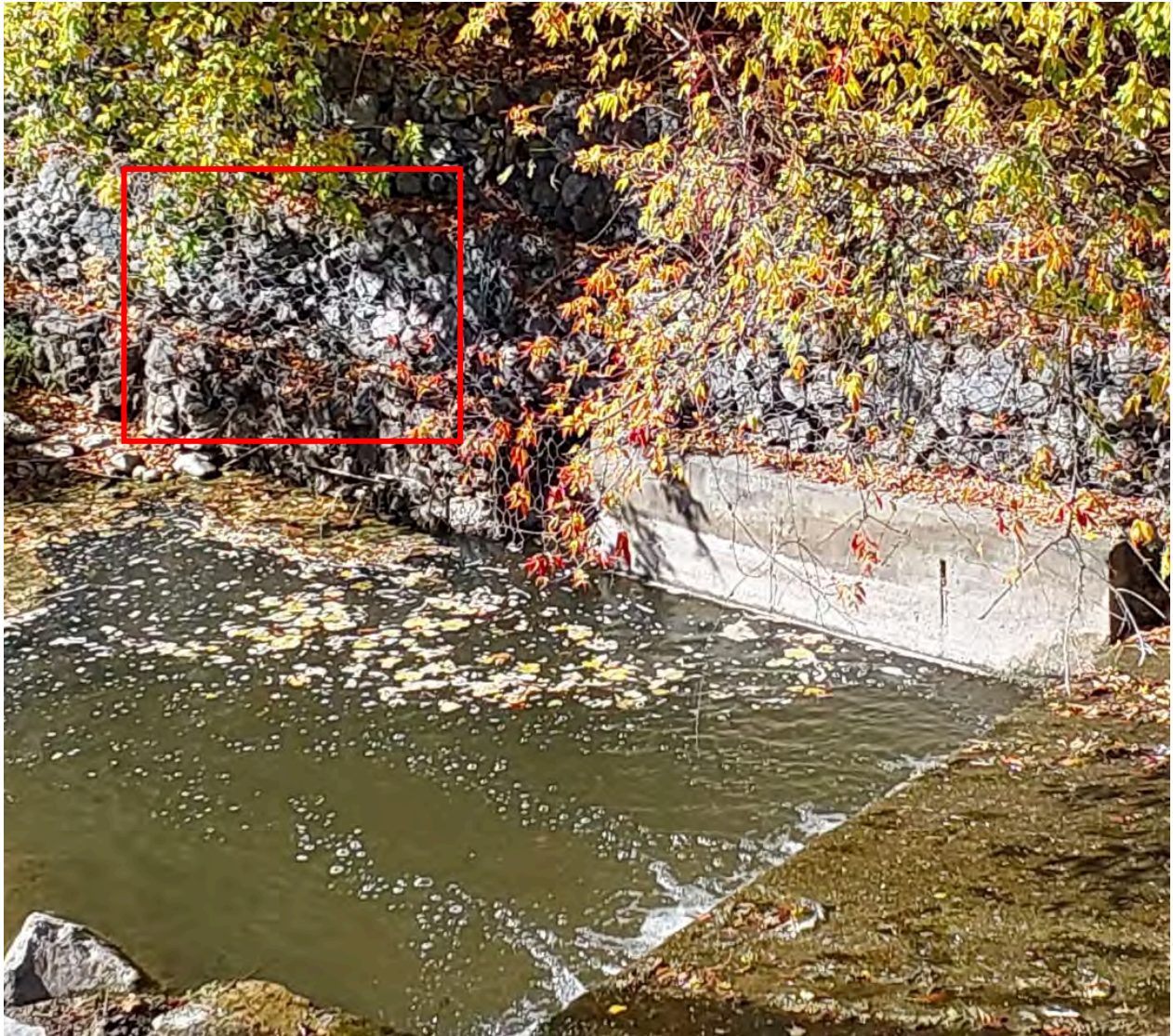
Figure 50: Missing stones from gabion basket on the north side of channel near weir dam, adjacent to 49 Mill Street.
