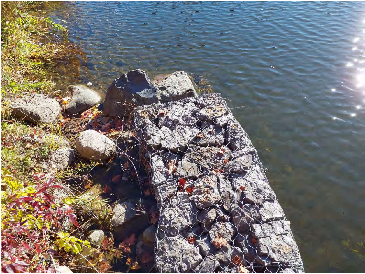
Figure 7: Southern side bank upstream of Dam. Gabion basket along edge of Dam pond.
