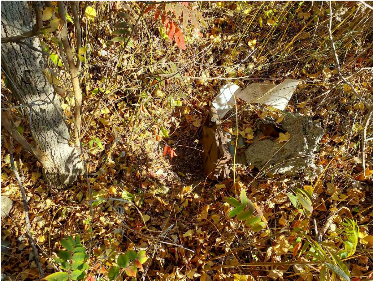
Figure 23: Clear flap gate 2 along north side of Douglas Road berm, with woody vegetation in flow path of flap gate.
