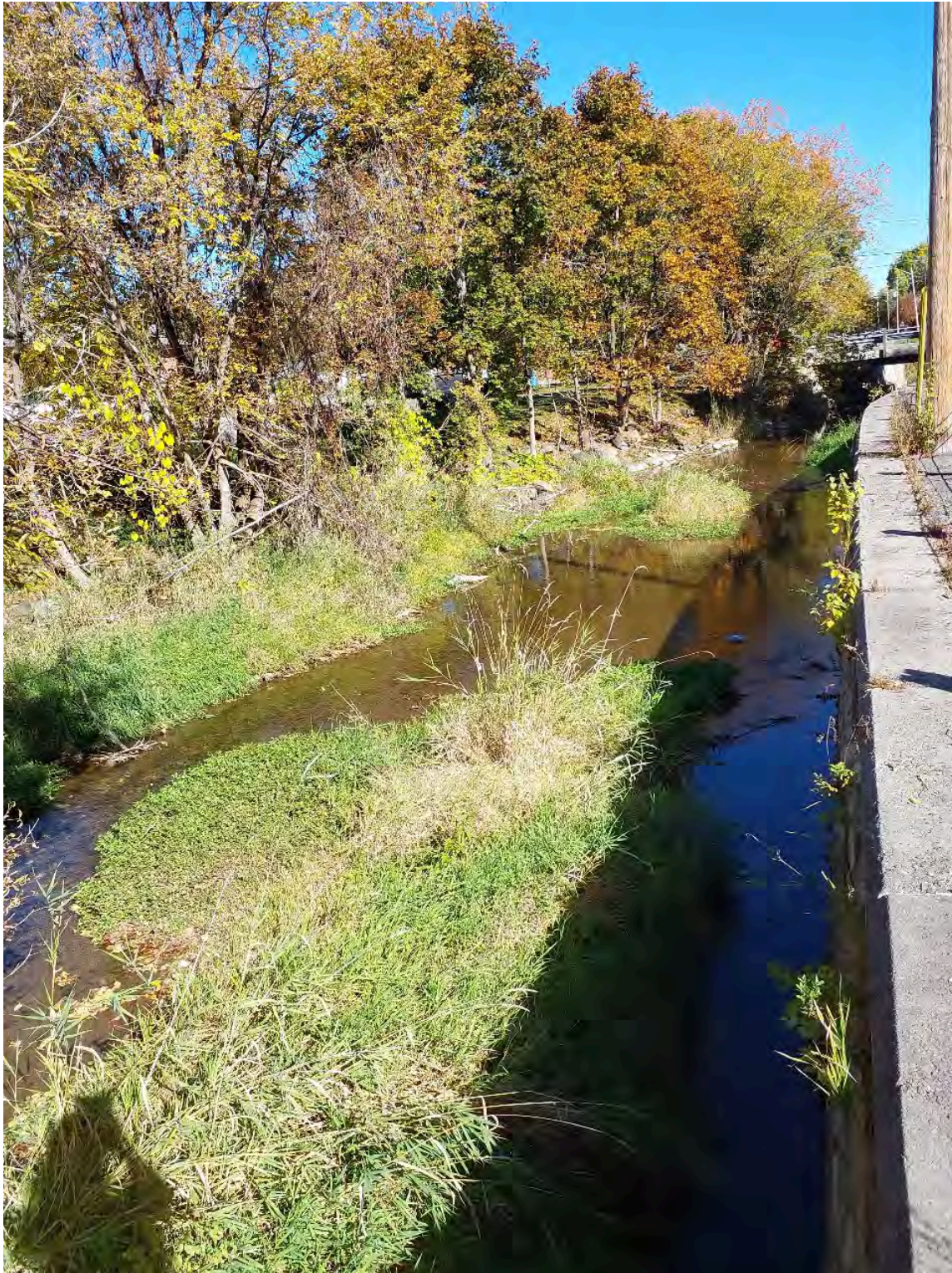
Figure 61: Sediment deposits and vegetation downstream of the Simpson Street bridge. Photo taken facing downstream from the bridge.
