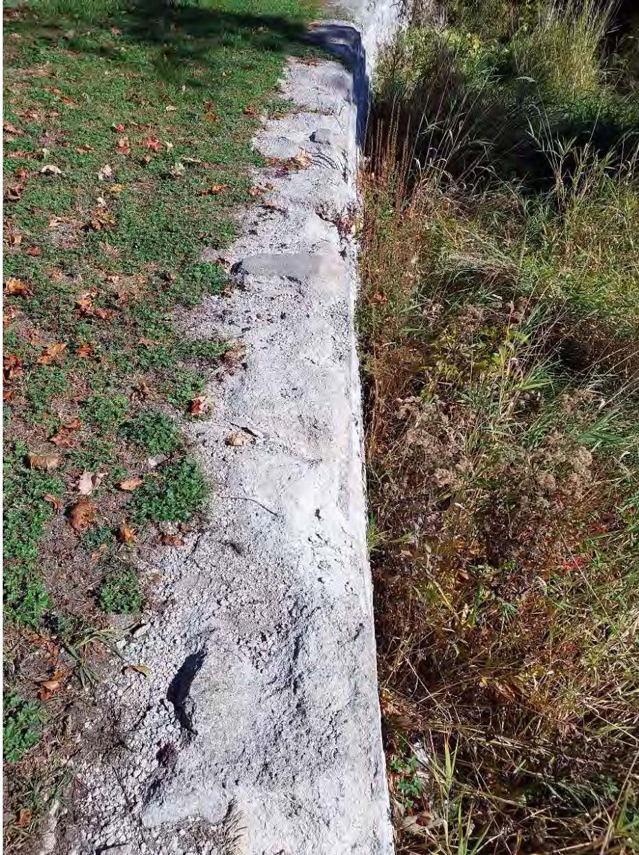
Figure 12: Durahold Block erosion along north side of LTC owned section of flood channel.
