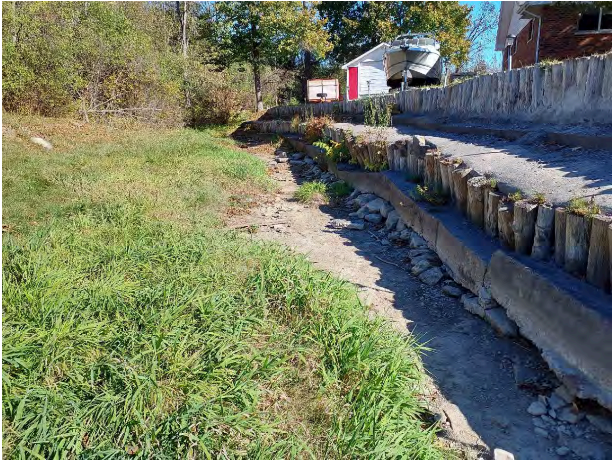
Figure 20: Sediment build-up with vegetation growth on the east side of box culvert at Peterson Street facing upstream.
