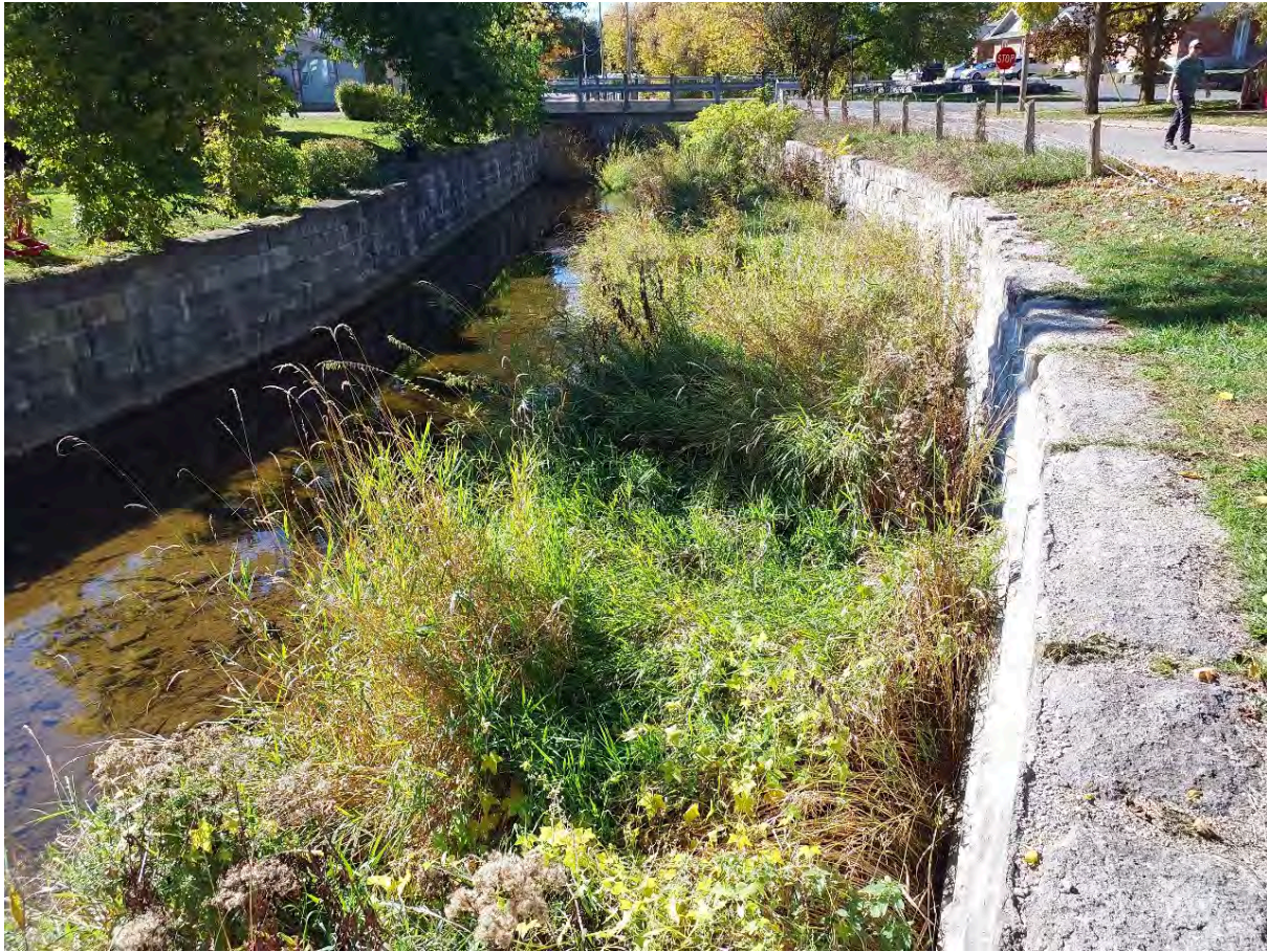
Figure 65: Upstream of Pellissier Street Bridge adjacent to Inkerman Street showing erosion of DuraHold blocks and excess sediment/ vegetation within the channel. Photo taken facing upstream.
