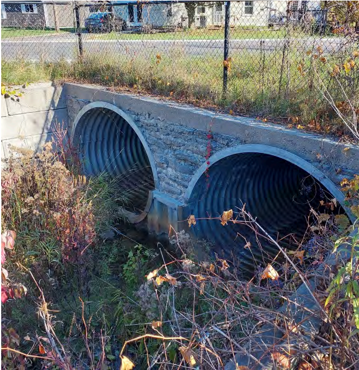
Figure 32: Double arch culvert under Wooler Road.
