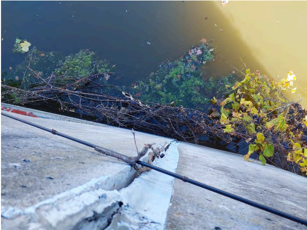
Figure 53: Crack repair in concrete wall along west side of channel upstream of weir.
