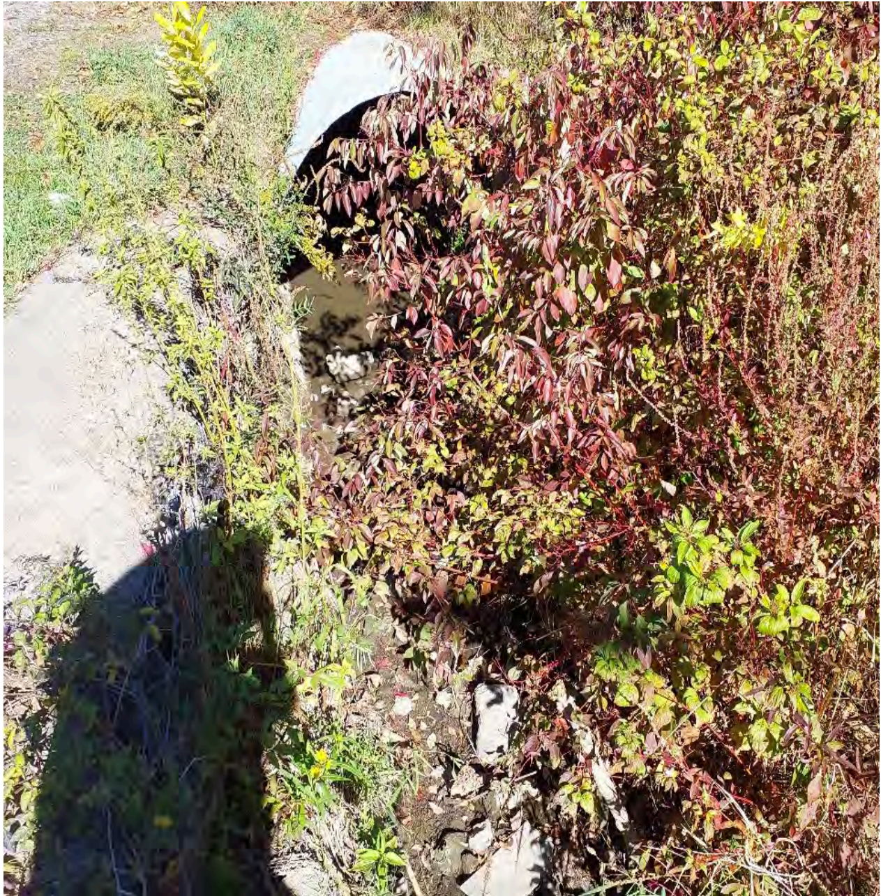
Figure 15: Byron Street – heavy vegetation downstream of culvert.
