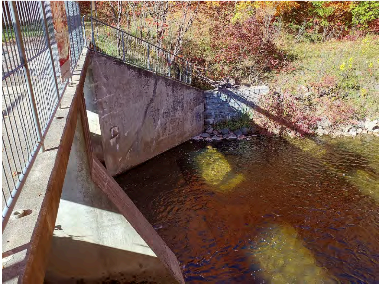
Figure 3: Northern wing wall on downstream side of Dam
