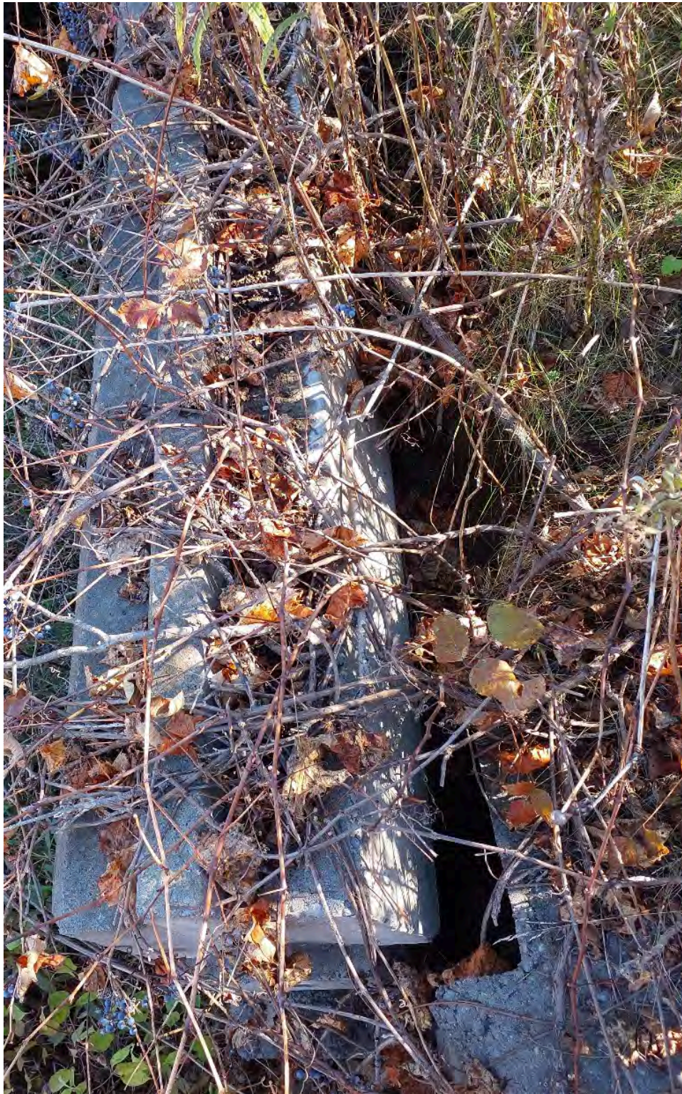
Figure 29: Wing wall on south side of Downstream Channel, downstream of Double Arch Culvert showing separation
