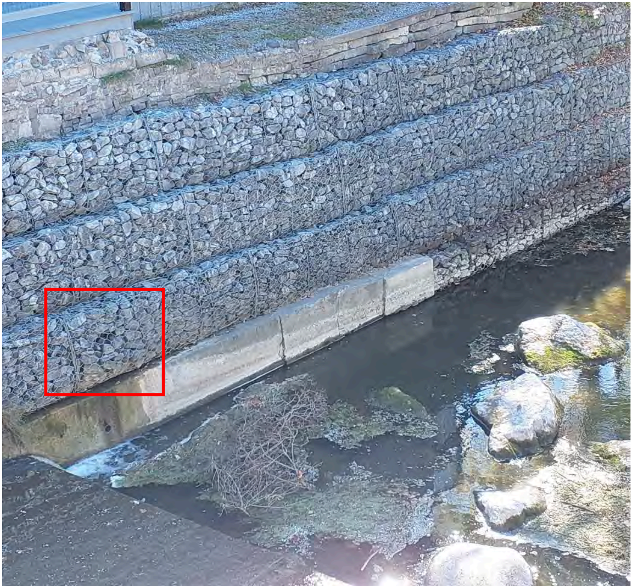
Figure 49: Missing stone from gabion basket on south side of channel near weir dam adjacent to 29 James Street.
