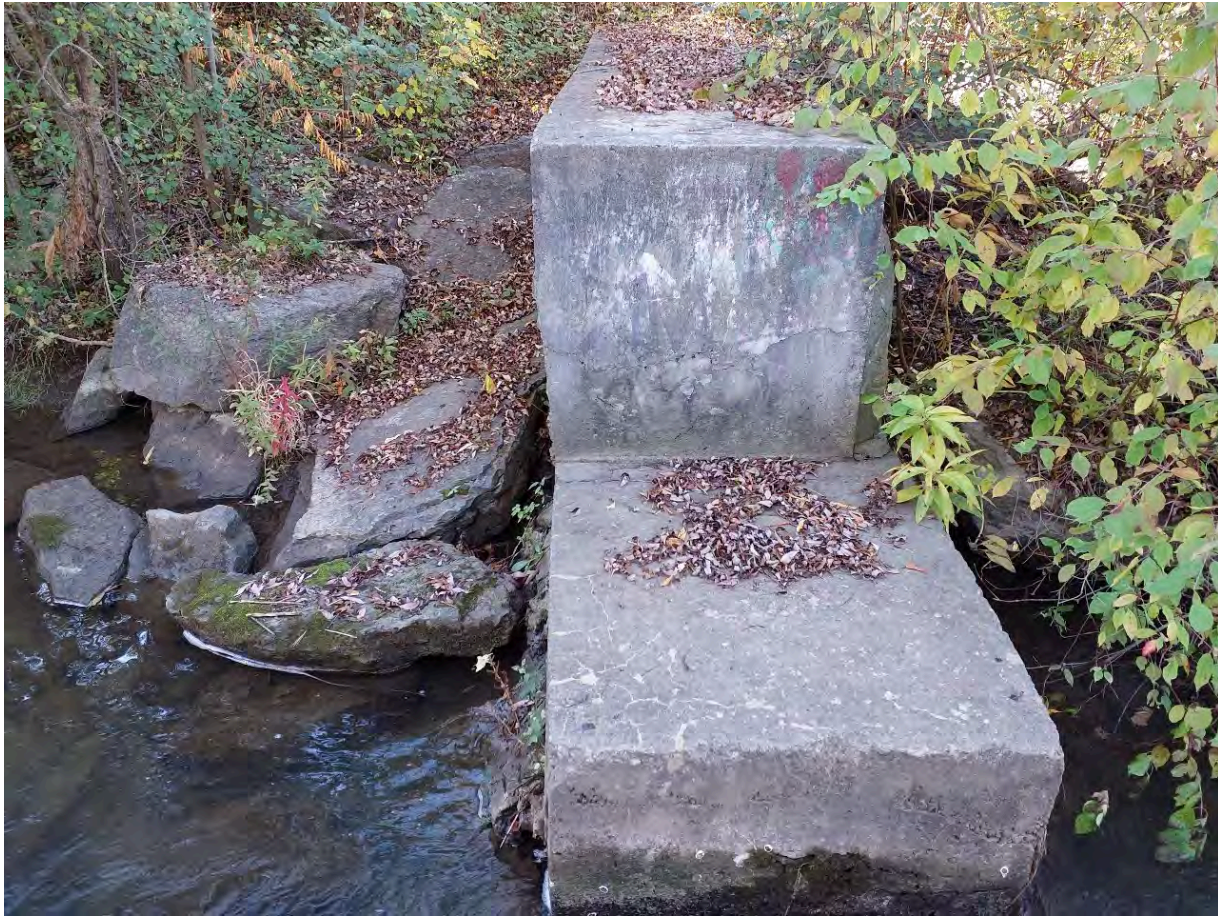
Figure 33: 2-Stage weir spalling on south side of watercourse.
