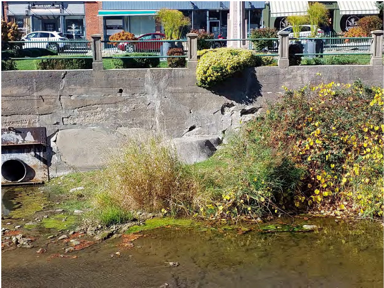
Figure 43: Additional view of identified cracks on north side of flood channel downstream of covered bridge.
