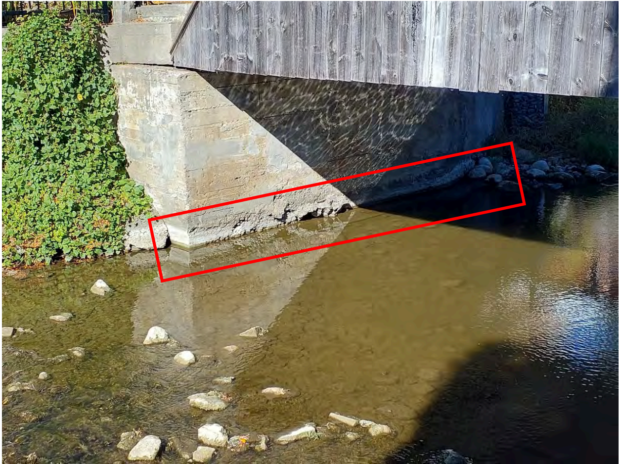
Figure 48: Erosion at toe of bridge abutment for north side of covered bridge along flood channel.
