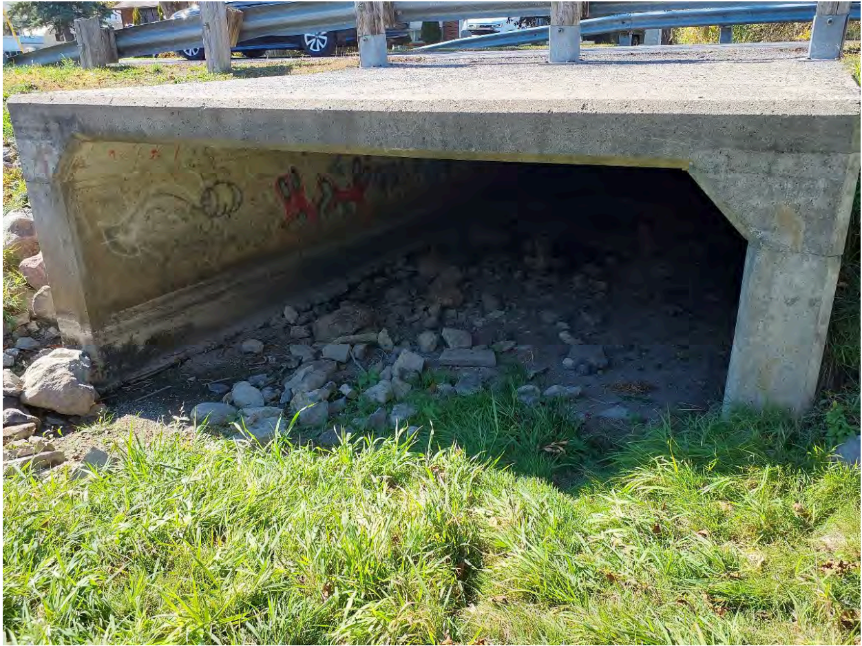
Figure 19: Sediment build-up with vegetation growth on the east side of box culvert at Peterson Street, facing downstream.
