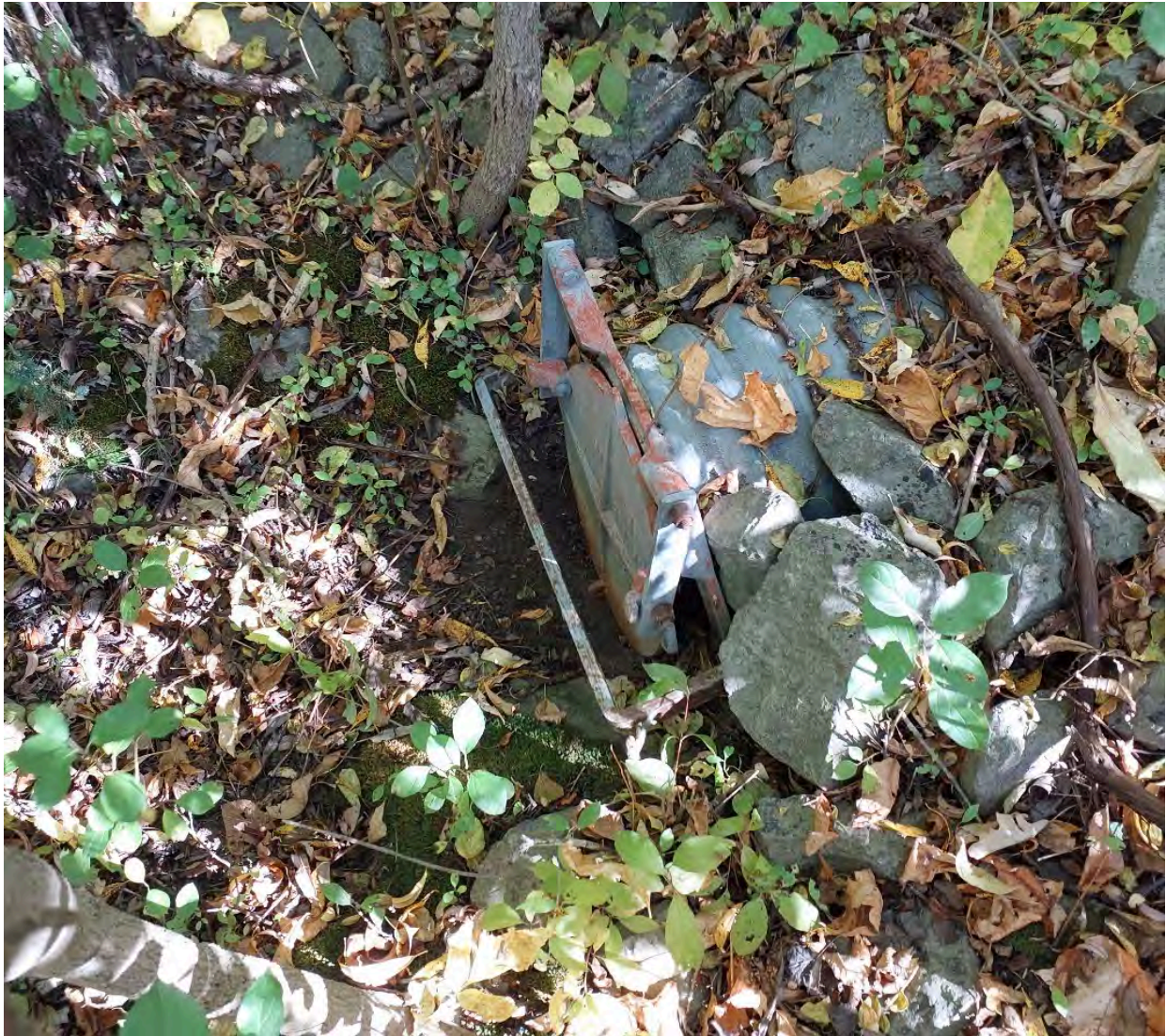
Figure 38: Cleared flap gate through berm on west side of berm.
