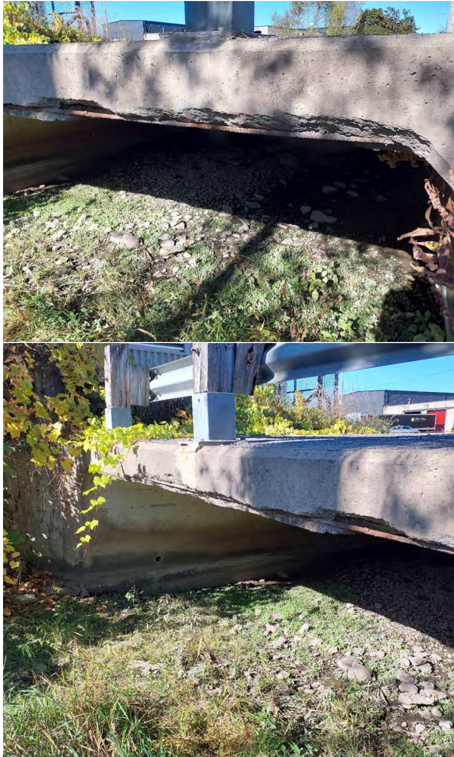
Figure 25/26: Spalling concrete with exposed rebar on downstream side of Foster Stearns Road box culvert.
