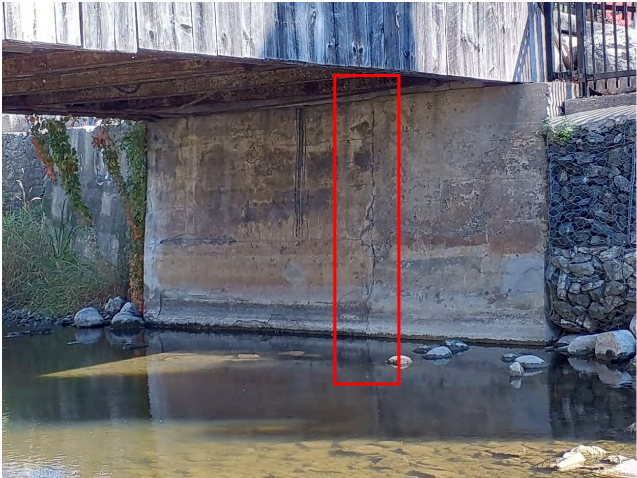
Figure 47: Vertical cracks on bridge abutment pf covered bridge on south wall of flood channel.
