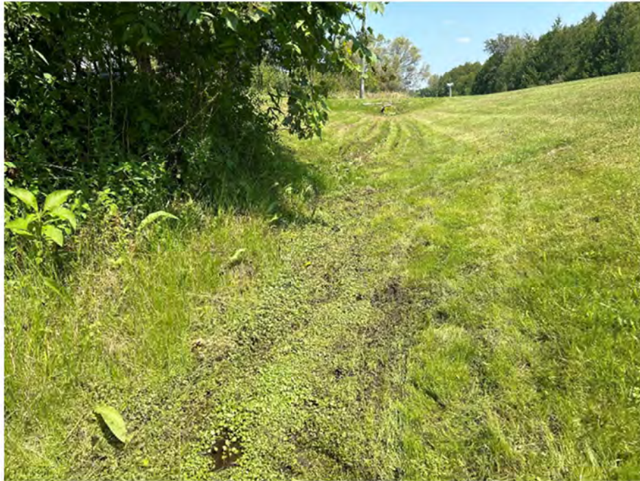
Photo 5 Looking east along ditch on north side of Shelter Valley Road, August 14, 2024.
