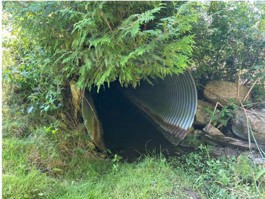
Photo 4 Looking downstream at culvert between roadside ditch and drainage feature, northeast of the Site, August 14, 2024.
