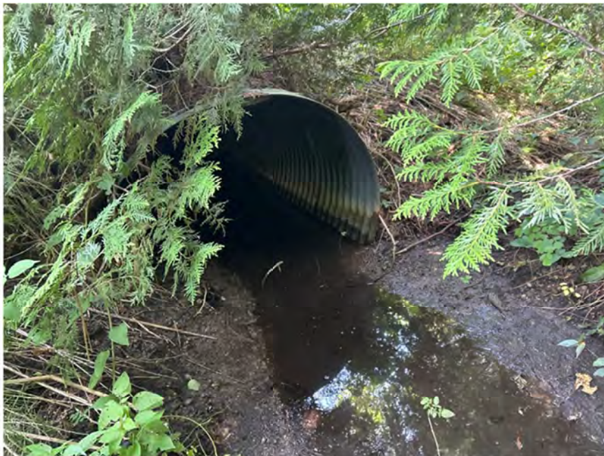
Photo 6 Culvert located on shelter valley road southeast of Site, August 14, 2024.
