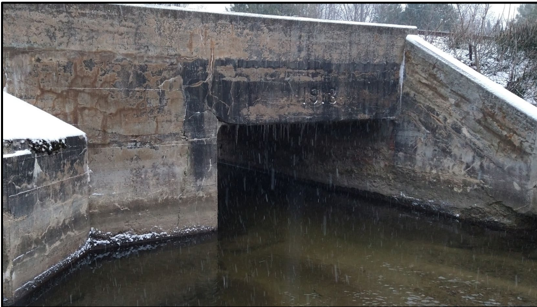
Figure 5-14: Image of Opening #2 for Butler Creek South Railway Crossing
