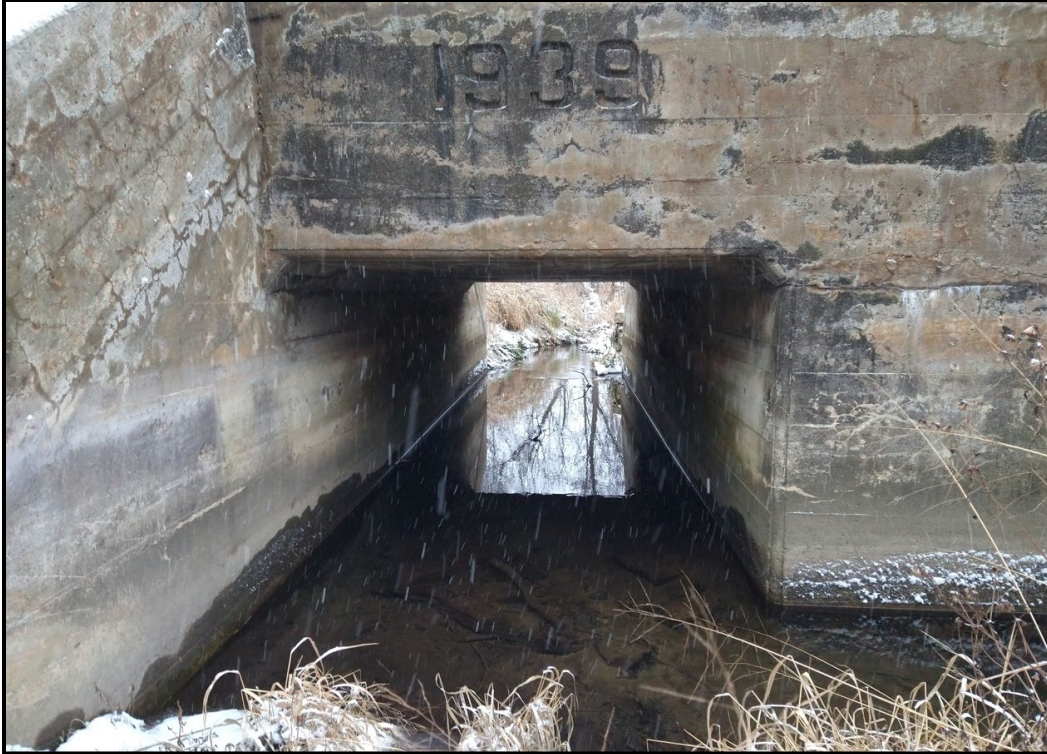
Figure 5-13: Image of Opening #1 for Butler Creek South Railway Crossing
