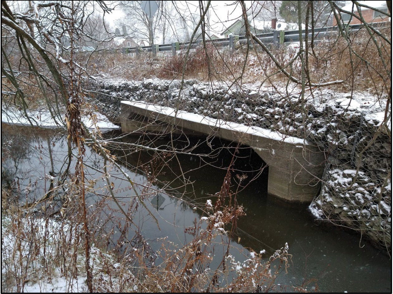
Figure 5-15: Ontario Street Opening Footing Box Culvert with 45 Degree Skew
