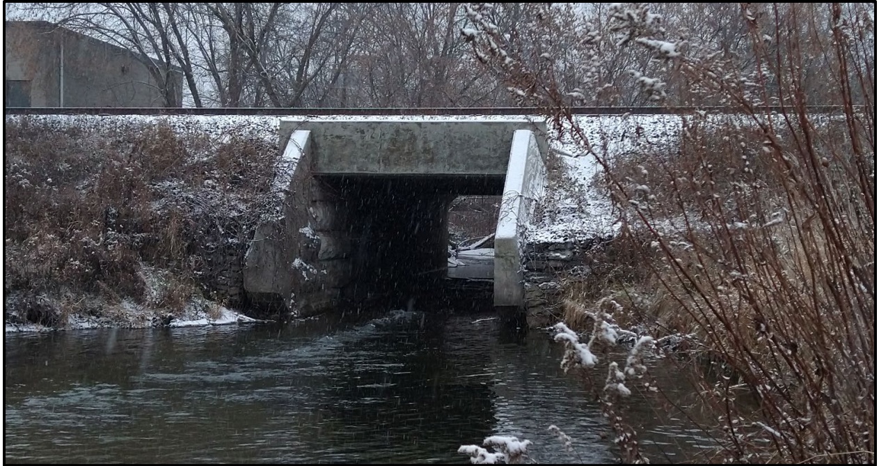
Figure 5-11: Image of Butler Creek North Railway Crossing
