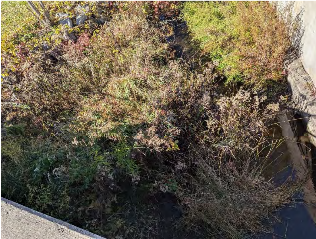
Figure 42: Flood channel facing downstream at Bay Street East culvert
