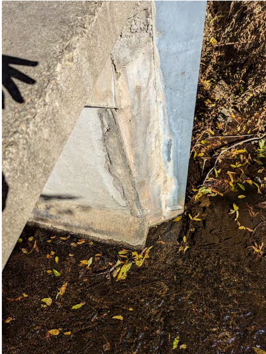
Figure 45: Water Street Twin Box Culvert eastern edge of upstream side
