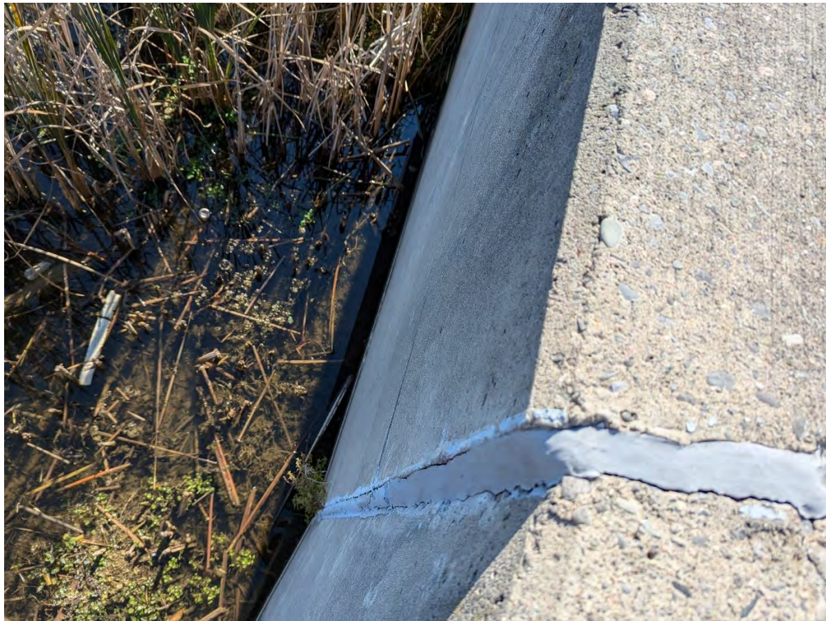
Figure 37: Repaired spalling on wall remaining unchanged since last inspection in 2023
