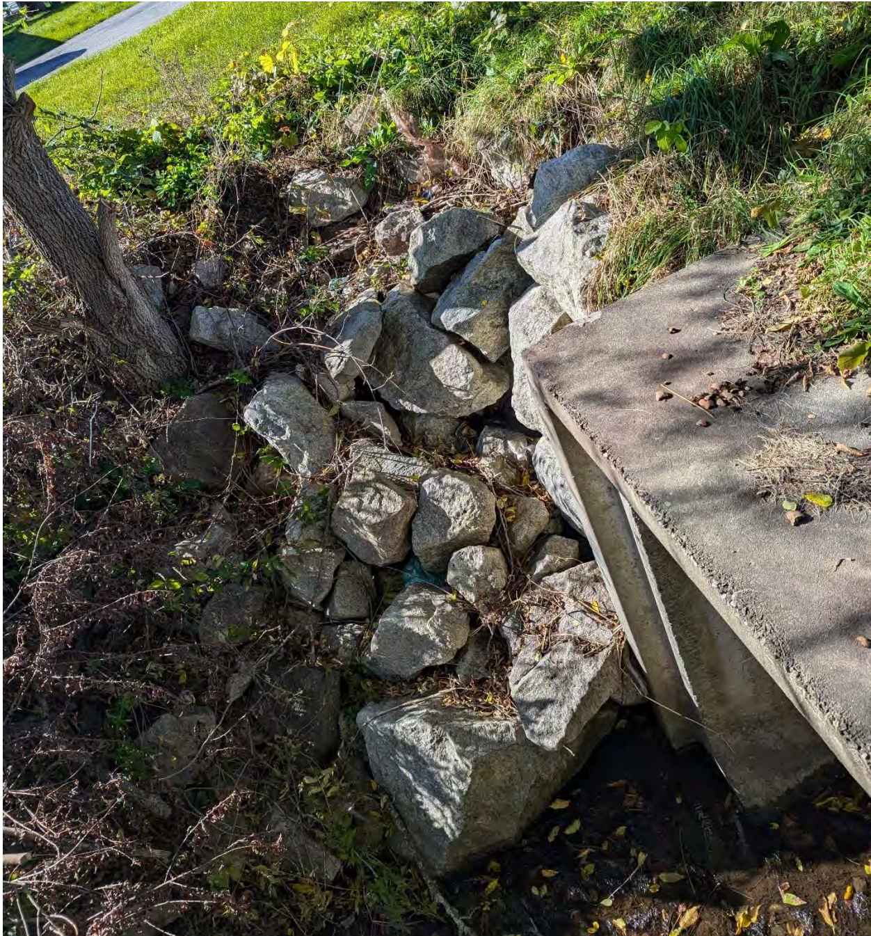
Figure 46: Water Street Twin Box Culvert western edge of upstream side
