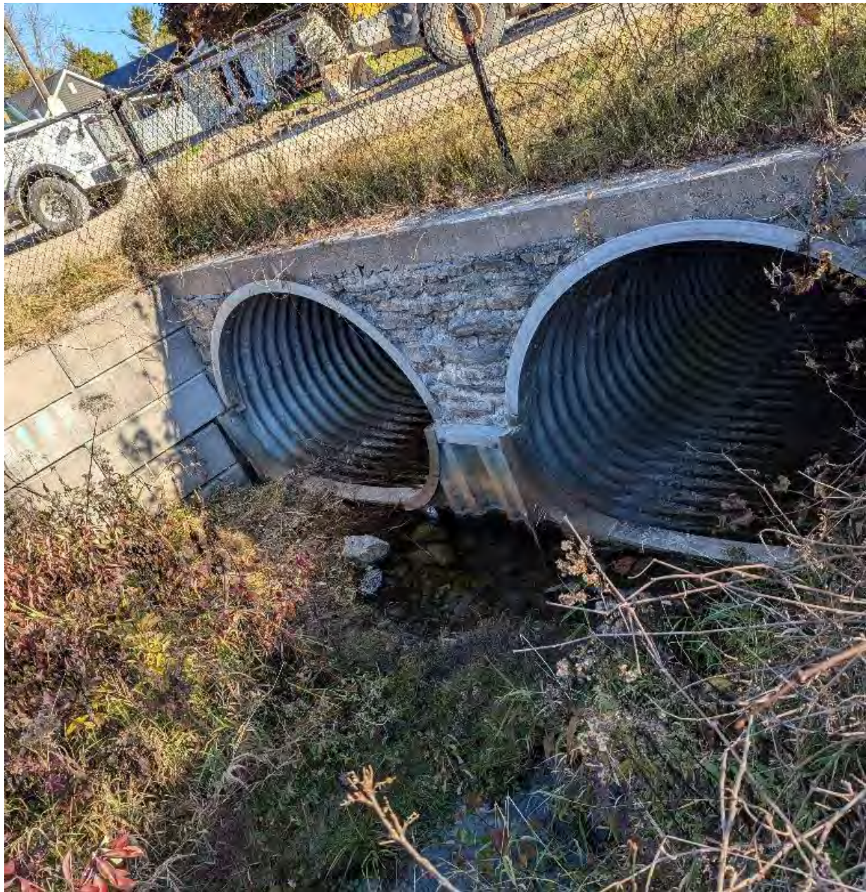
Figure 28: Double arch culvert under Wooler Road
