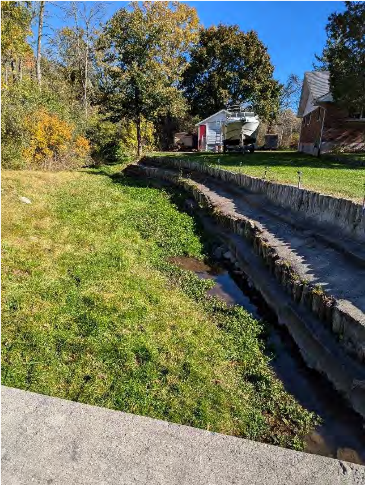
Figure 17: Sediment build-up on the east side of box culvert at Peterson Street facing upstream
