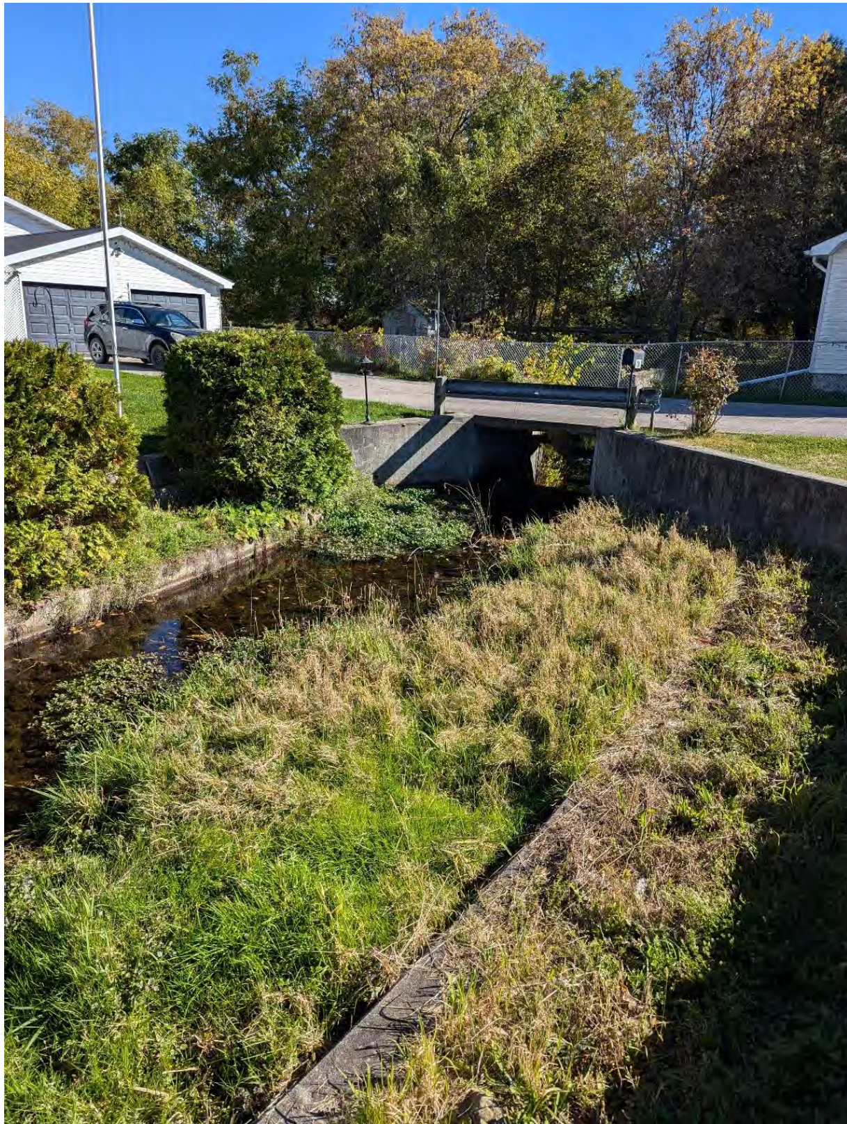
Figure 43: Channel crossing and vegetation within the flood channel adjacent to Park Street
