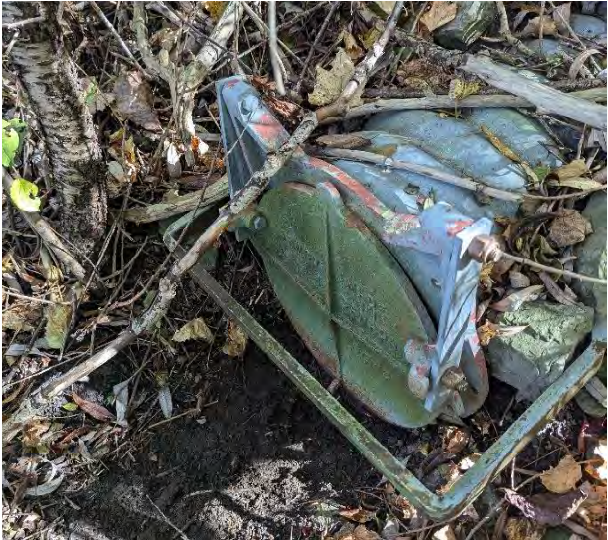
Figure 30: Cleared flap gate through berm
