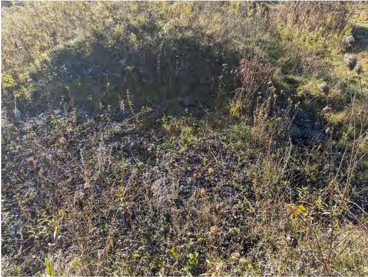
Figure 24: Minimal Vegetation on Berm Spillway
