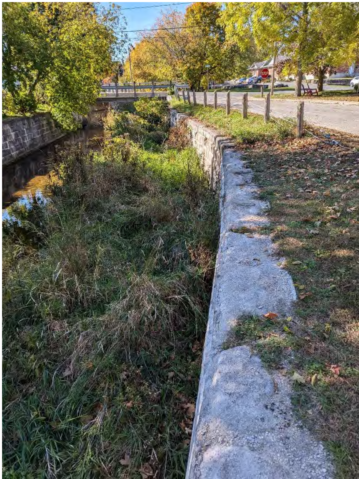
Figure 49: Upstream of Pellissier Street Bridge adjacent to Inkerman Street
