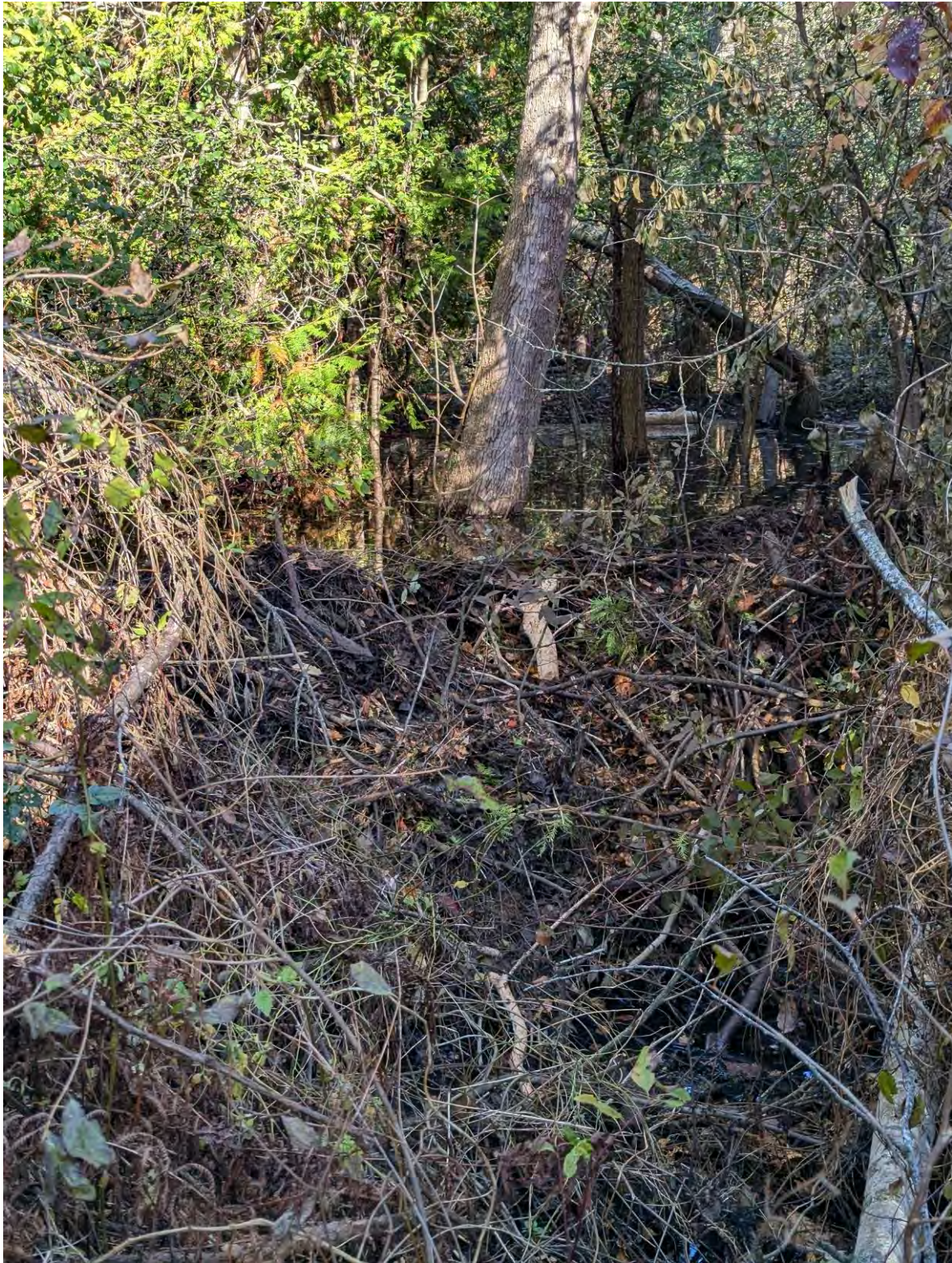
Figure 10: Downstream side of beaver dam
