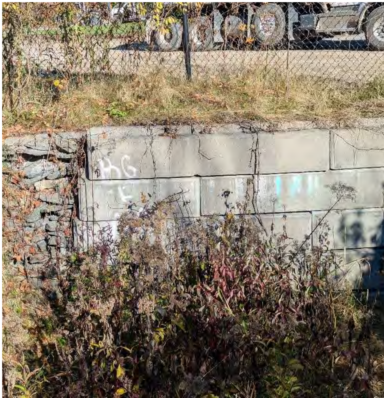
Figure 27: Wing wall (north side) downstream of the Double Arch culvert under Wooler Road
