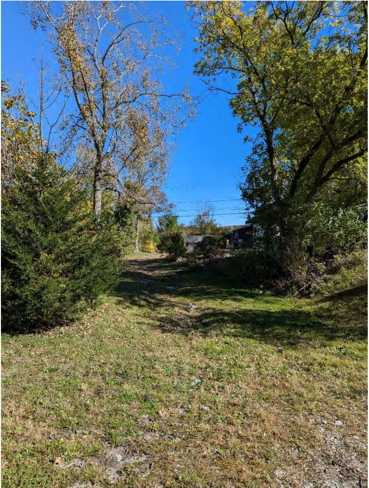
Figure 11: Main spillway between golf course and spillway bridges
