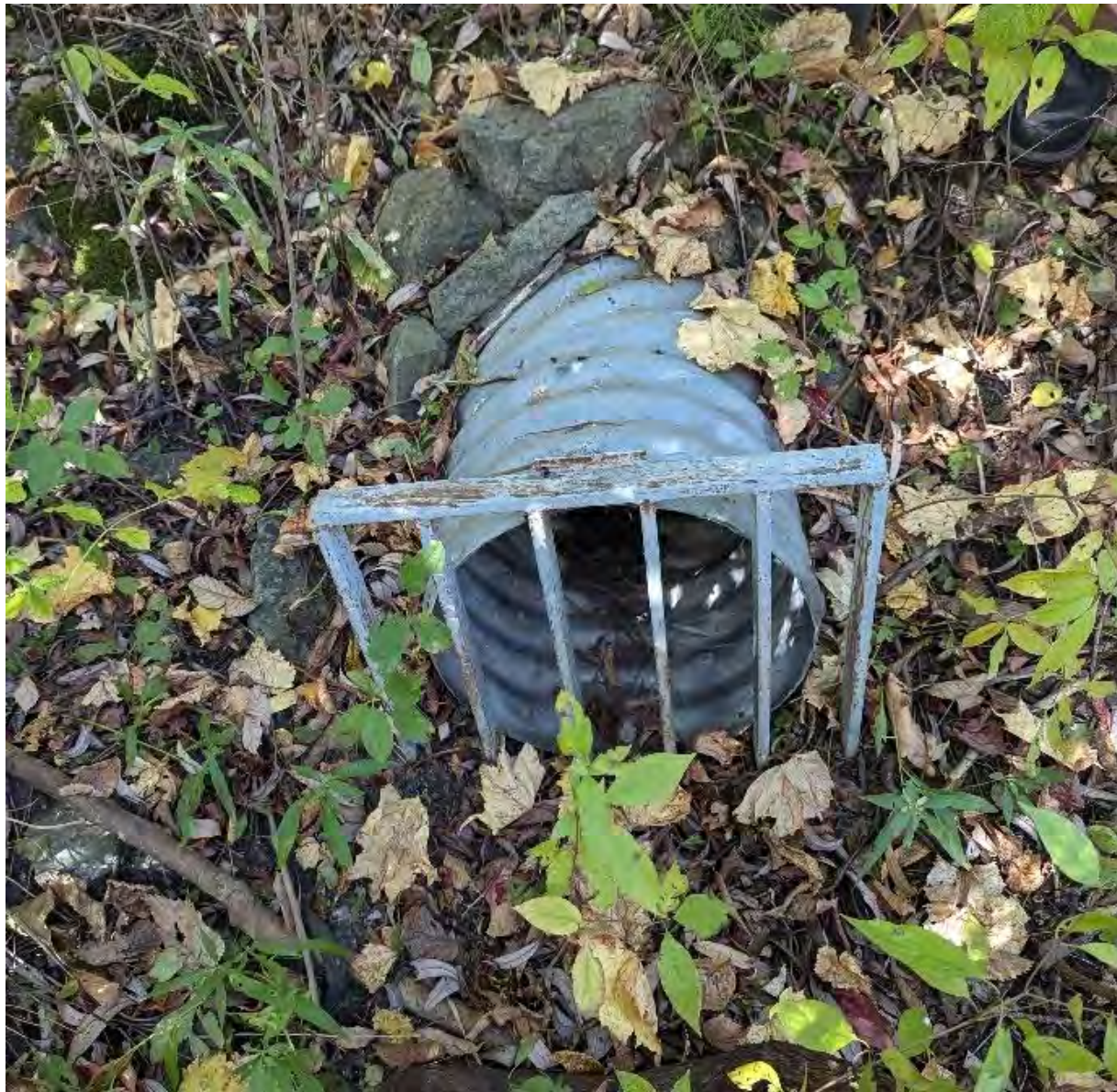
Figure 31: Inlet to flap gate through berm
