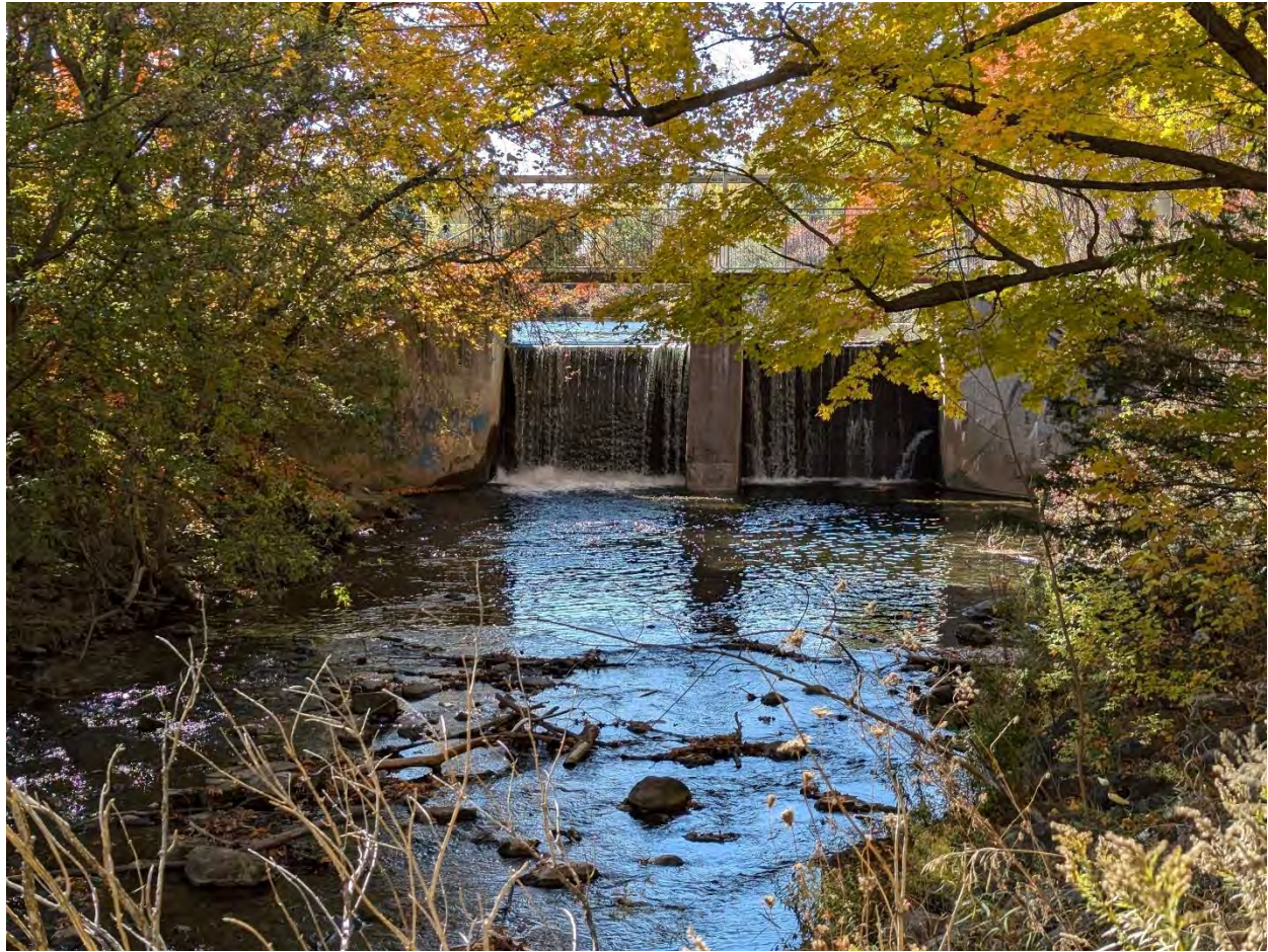
Figure 1: Downstream side of Dam
