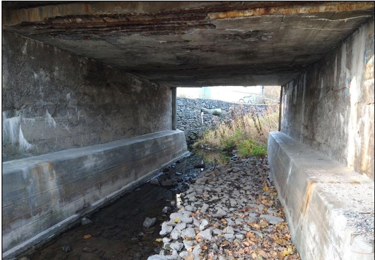
Figure 5-29: View of Bridge Opening at Front Street Diversion Channel Crossing
