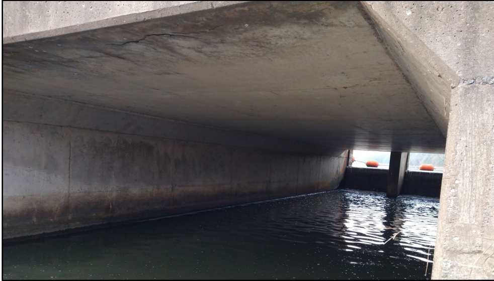
Figure 5-12: View from Downstream Side of Tremur Lake Dam Opening
