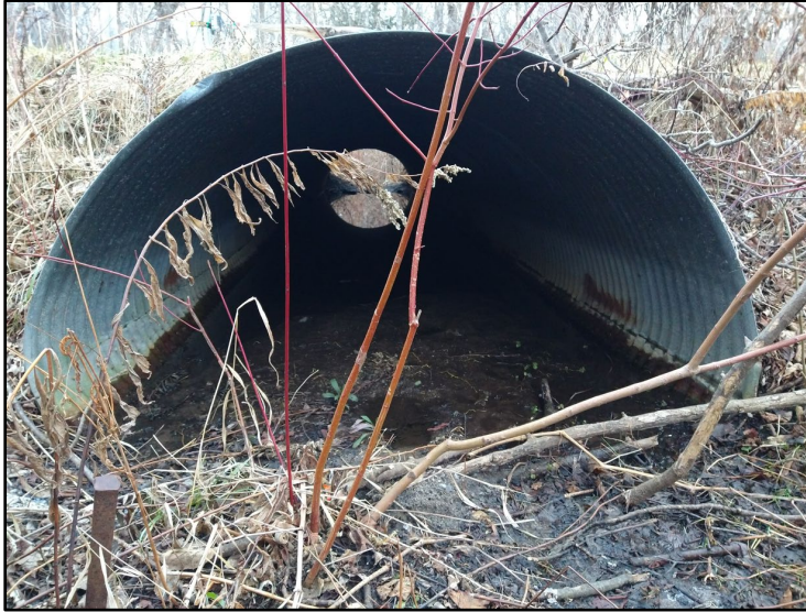
Figure 6-11: March Street Spill Culvert
