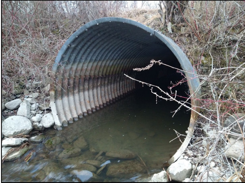
Figure 5-9: Culvert Opening for Access Road Crossing
