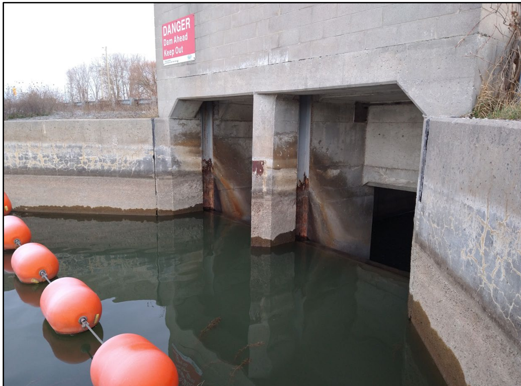
Figure 5-11: View of Upstream Side of Tremur Lake Dam Opening
