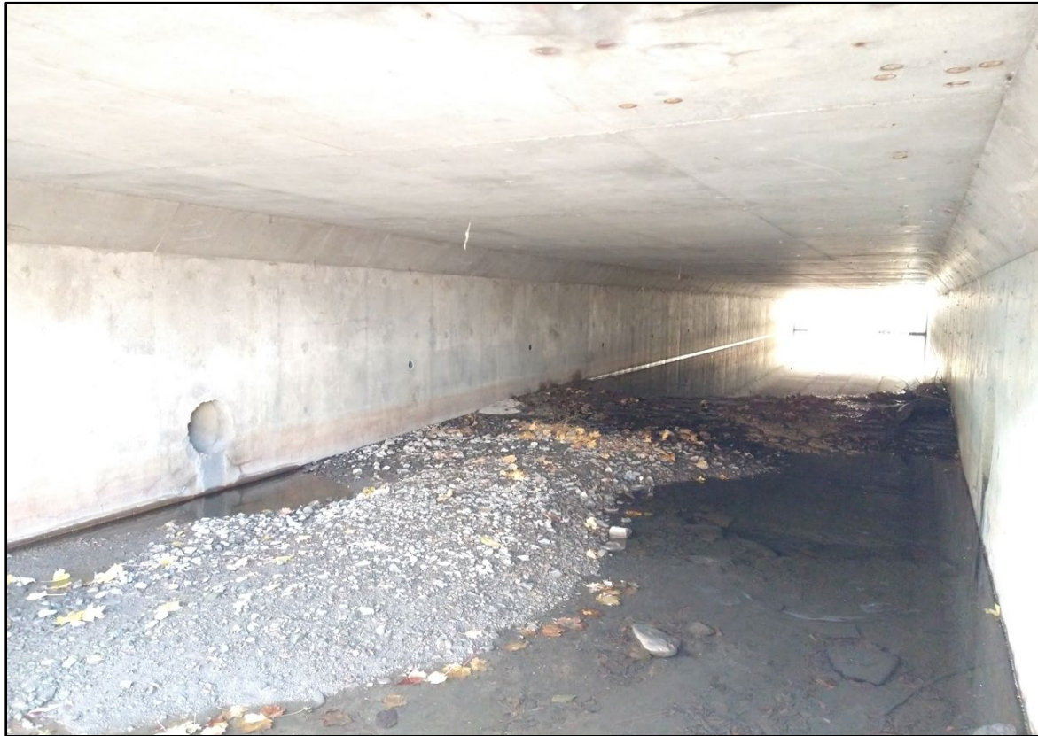
Figure 5-30: View of Culvert Opening at Front Street Diversion Channel Crossing
