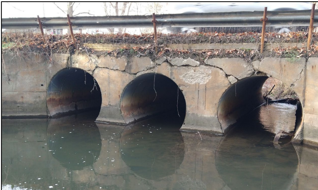
Figure 5-16: Elevation View of 2 nd Dug Hill Road Culverts
