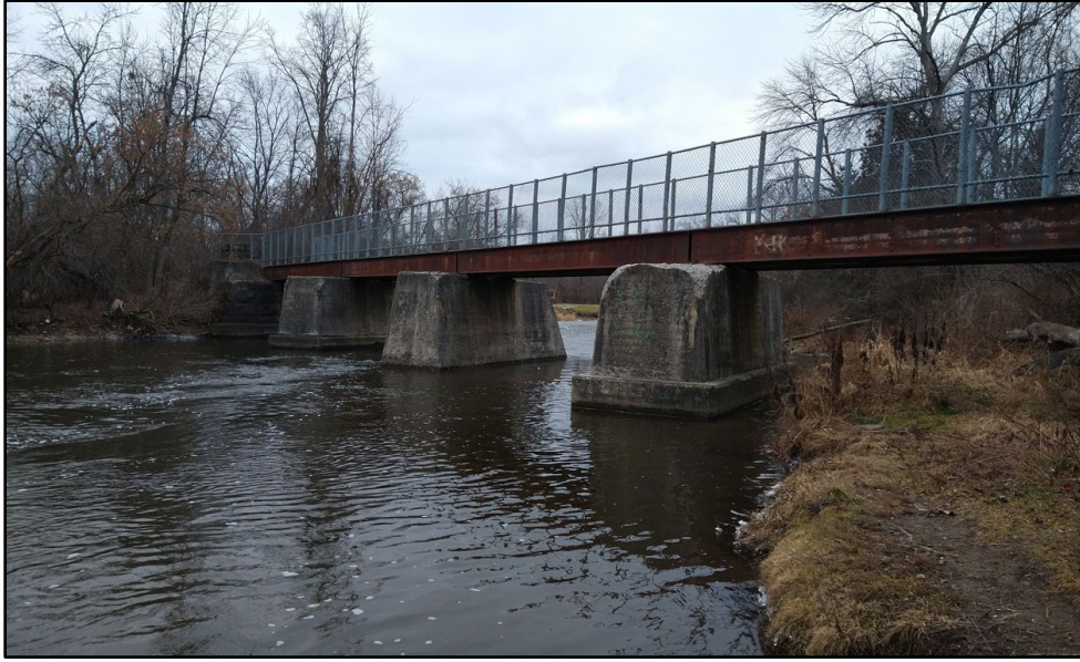
Figure 6-5: Elevation View of Old Railway Bridge
