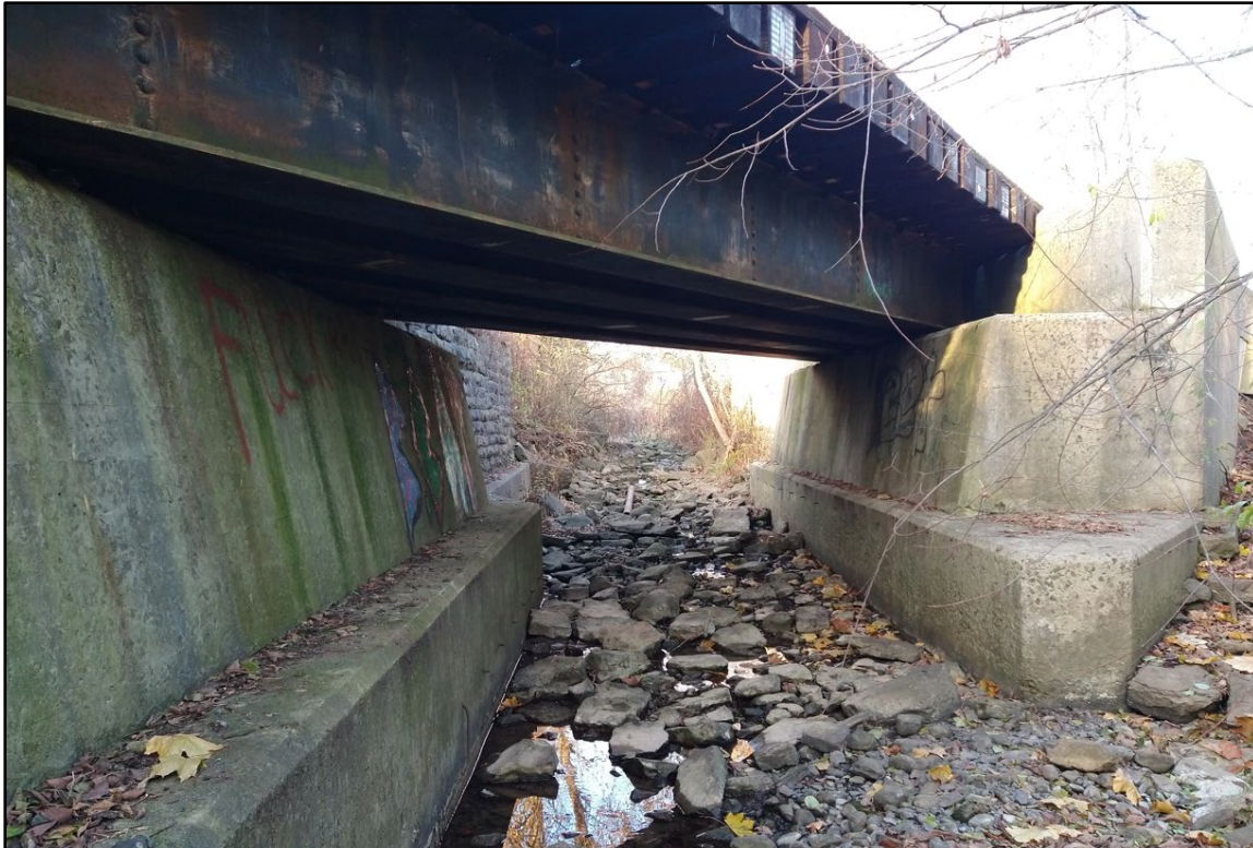
Figure 5-26: View of Bridge Opening at Old Railway Crossing of Diversion Channel
