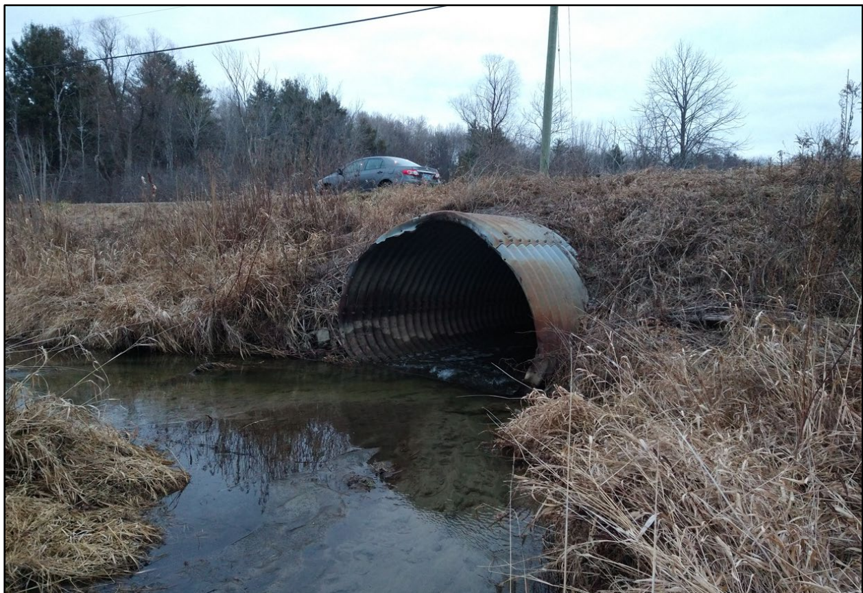
Figure 5-6: Elevation View of Tate Road Culvert Crossing
