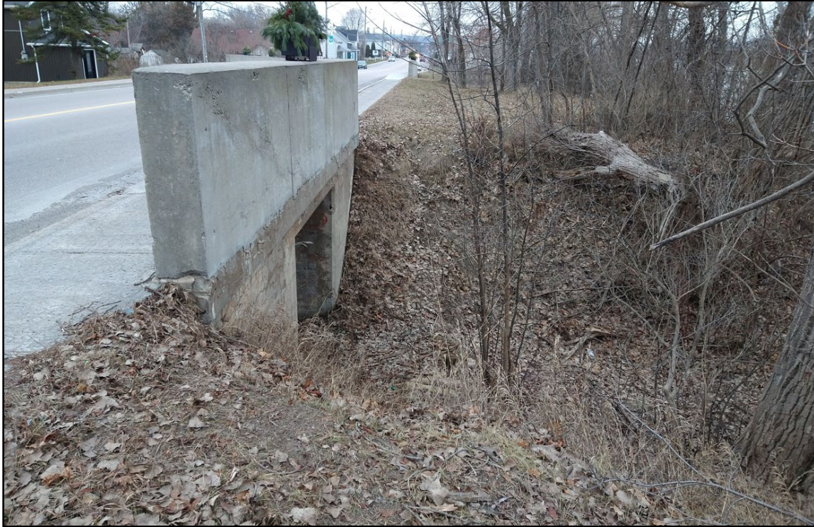
Figure 6-15: Middle Spill Crossing at South Trent Street
