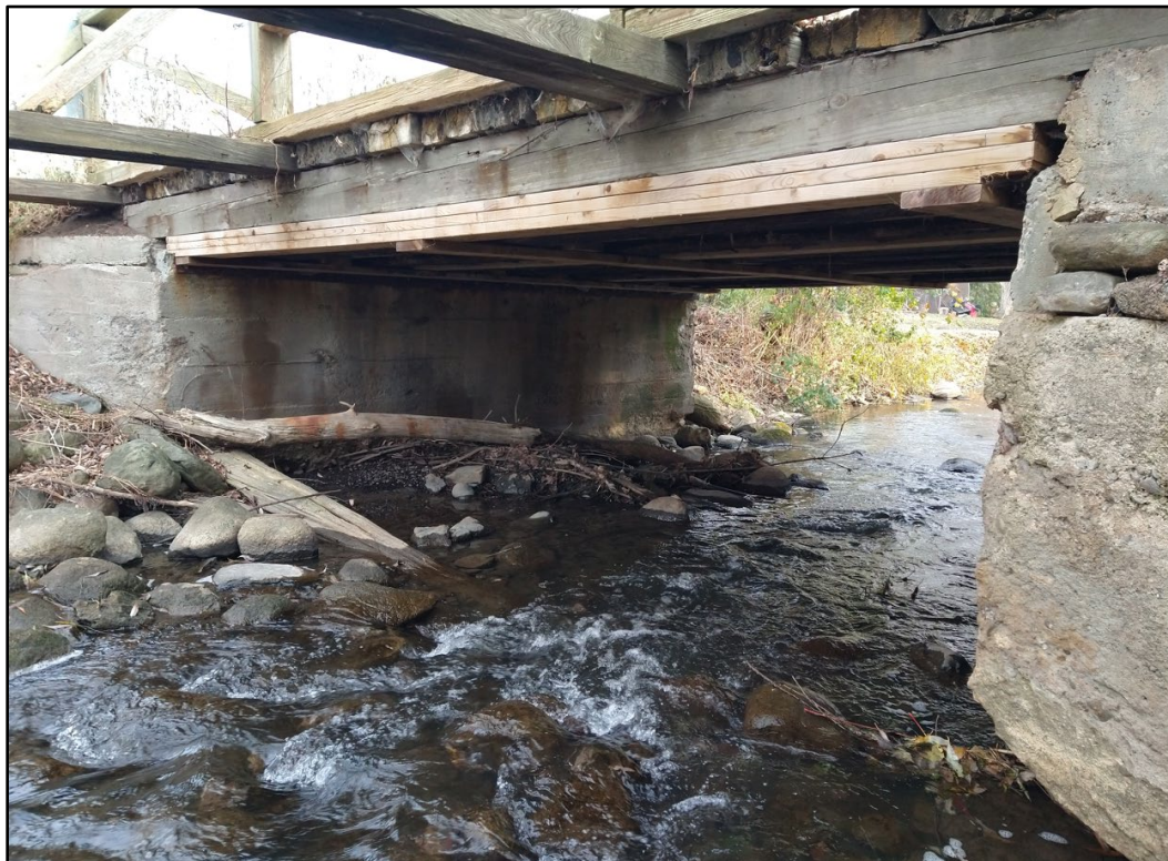
Figure 5-15: Elevation View of Hill Road Bridge
