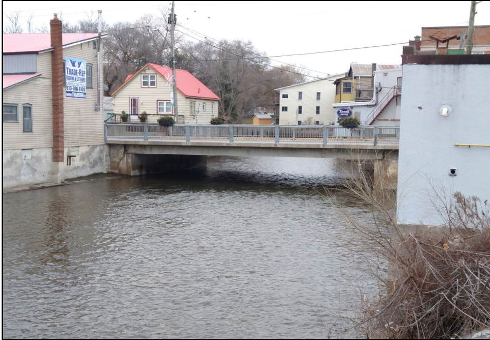
Figure 6-8: Crossing #2 - South Trent Street Bridge Outlet to Trent River
