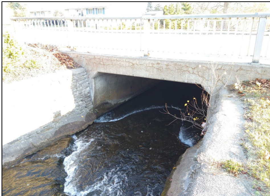
Figure 5-22: Water Street (A) Crossing
