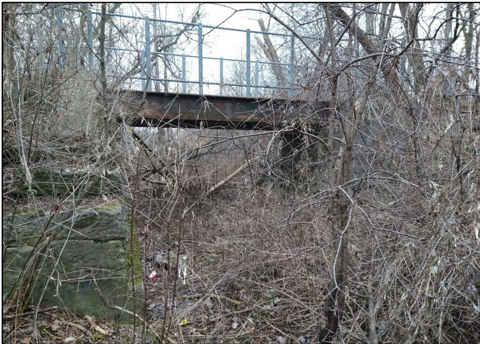
Figure 6-6: Old Railway Bridge Overflow Opening
