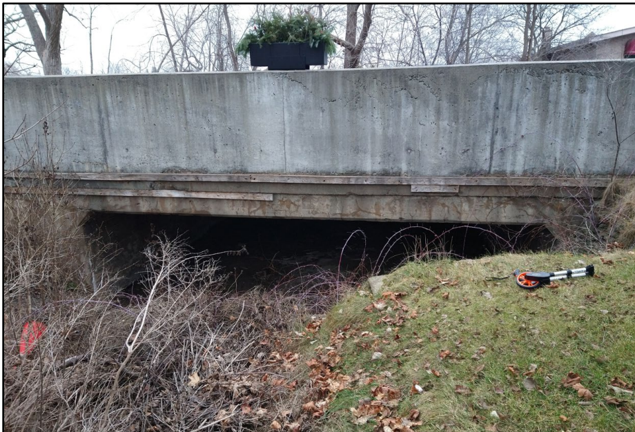
Figure 6-16: South Spill Crossing at South Trent Street
