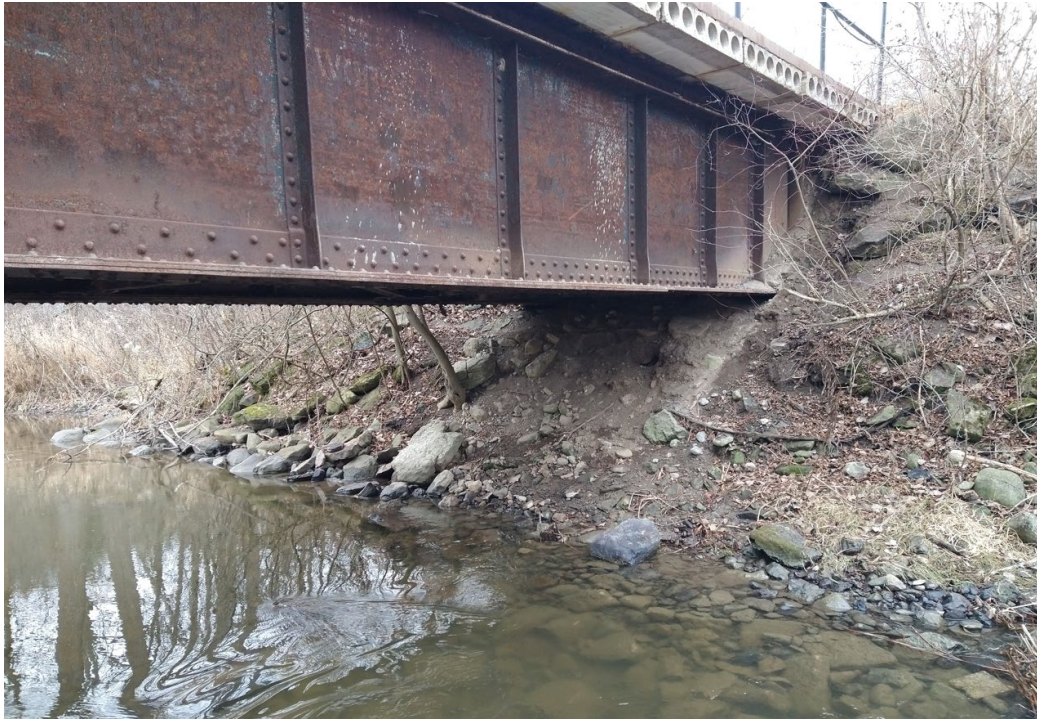
Figure 5-12: Image of Sloping Ground at Bridge Opening Simulating a Sloping Abutment
