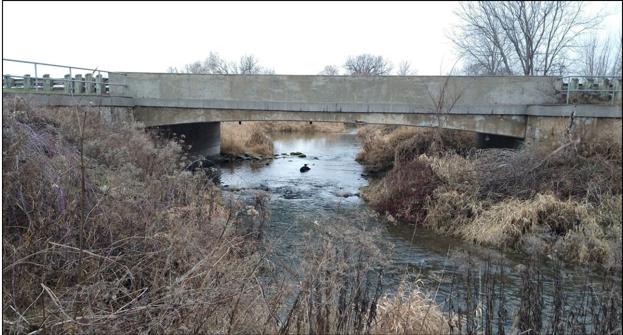
Figure 5-28: Elevation View of Bridge at Frankford Stirling Road
