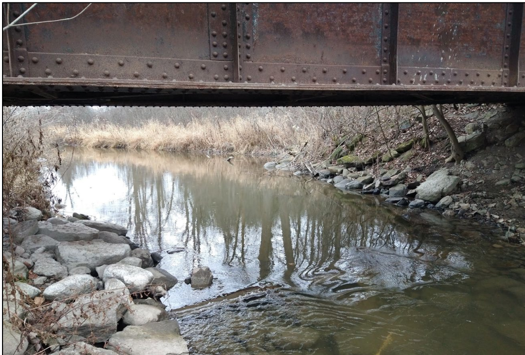
Figure 5-11: Image of Crossing to Aggregate Site
