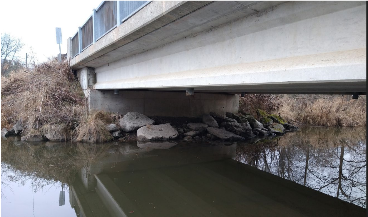
Figure 5-8: Image of Evergreen Road Bridge Opening
