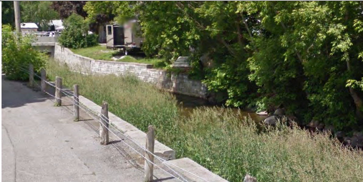
Figure 39: North Bank DuraHold retaining wall transition to river rock protection
