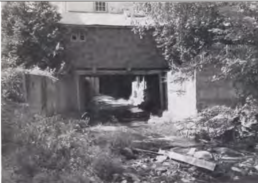
Figure 6: By-Pass Channel (Secondary Spillway) under 2 roads and houses
