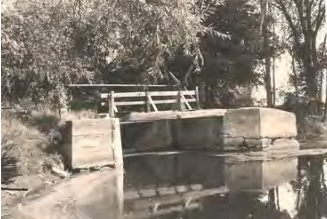
Figure 5: Photo of "Old" Warkworth Dam – 1967
