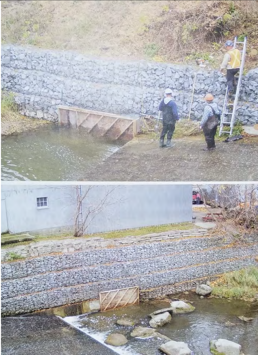
Figure 33: Concrete work for failing gabions in 2007
