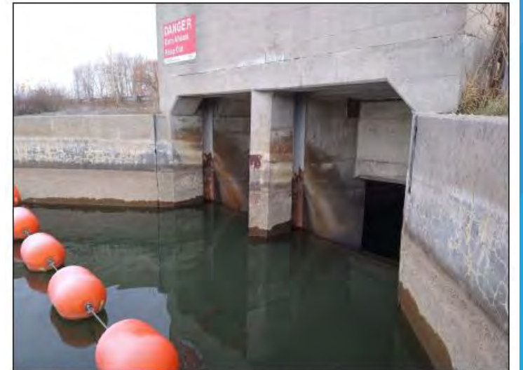
Figure 5-11: View of Upstream Side of Tremur Lake Dam Opening
