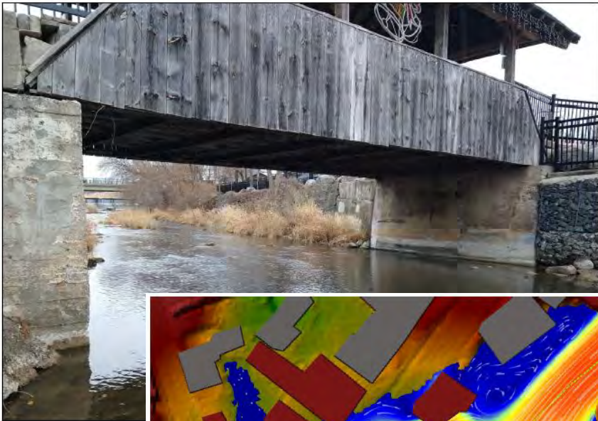
Figure 5-21: Image of Bridge
