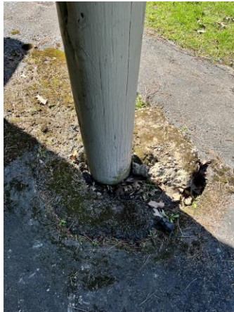
Asphalt and fill around post
