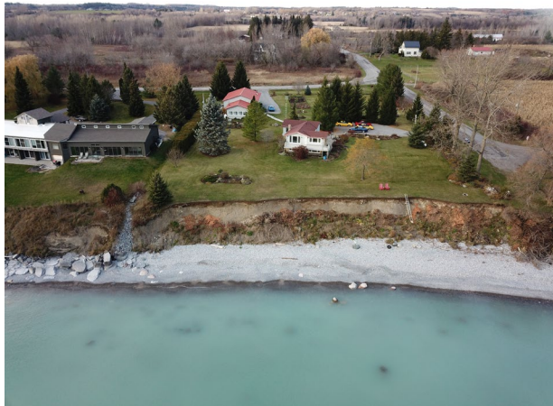
Eroding Bluff Shoreline, Victoria Beach
