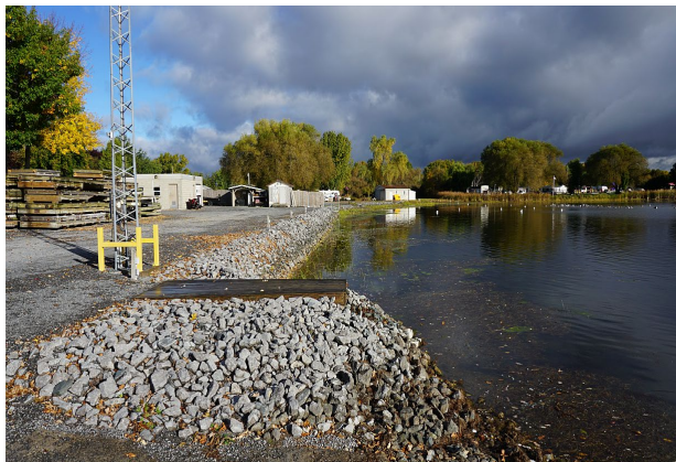
Armoured Shoreline at Trailer Park
