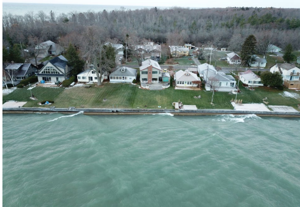
Concrete Seawalls, Presqu’ile Backside
