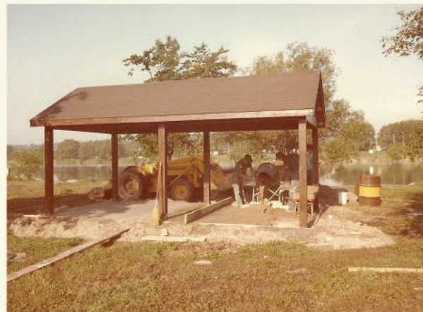
New Picnic Shelter for Glen Miller Conservation Area
