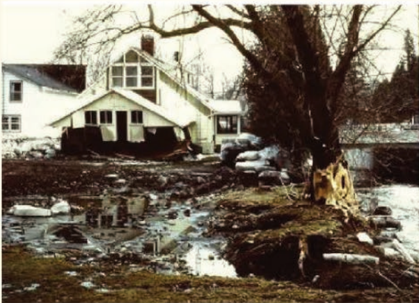
Warkworth Flood Damage (March 1980)
