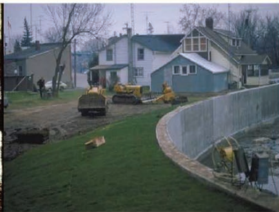
Construction of Floodwall (1982)
