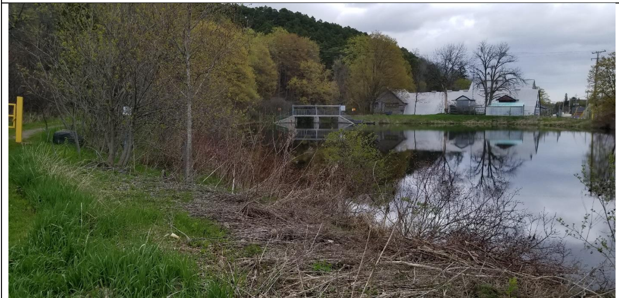
View of pond – summer operation level
